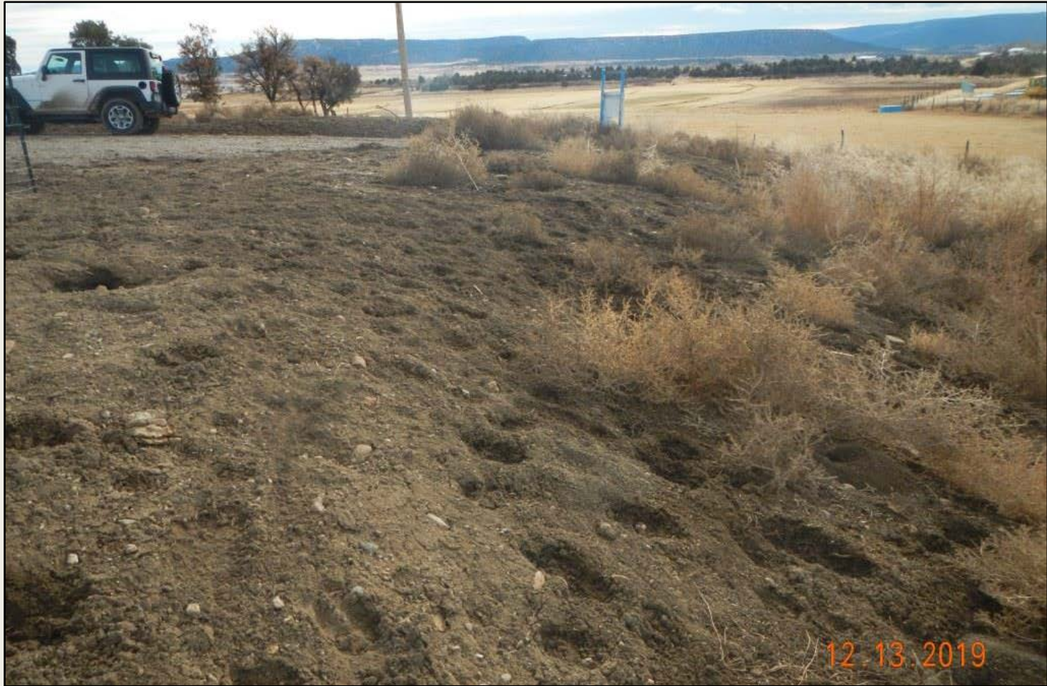
Photo 4. View of area in the western fill slope where revegetation is failed and revegetation/stabilization measures are needed.
