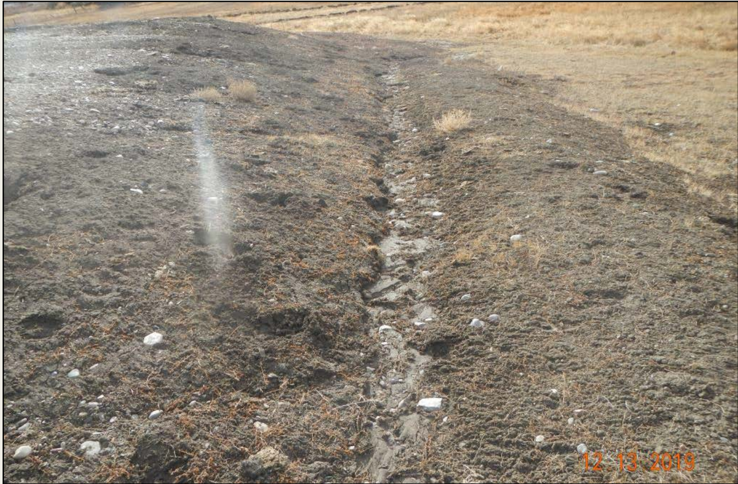
Photo 3. View of diversion and bare soils within the northwestern project area that are not stabilized.
