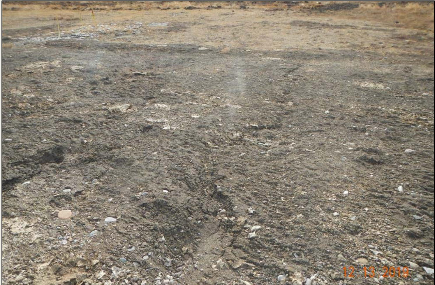
Photo 5. View of rilling and bare soils within the southwestern project area needing stabilization.
