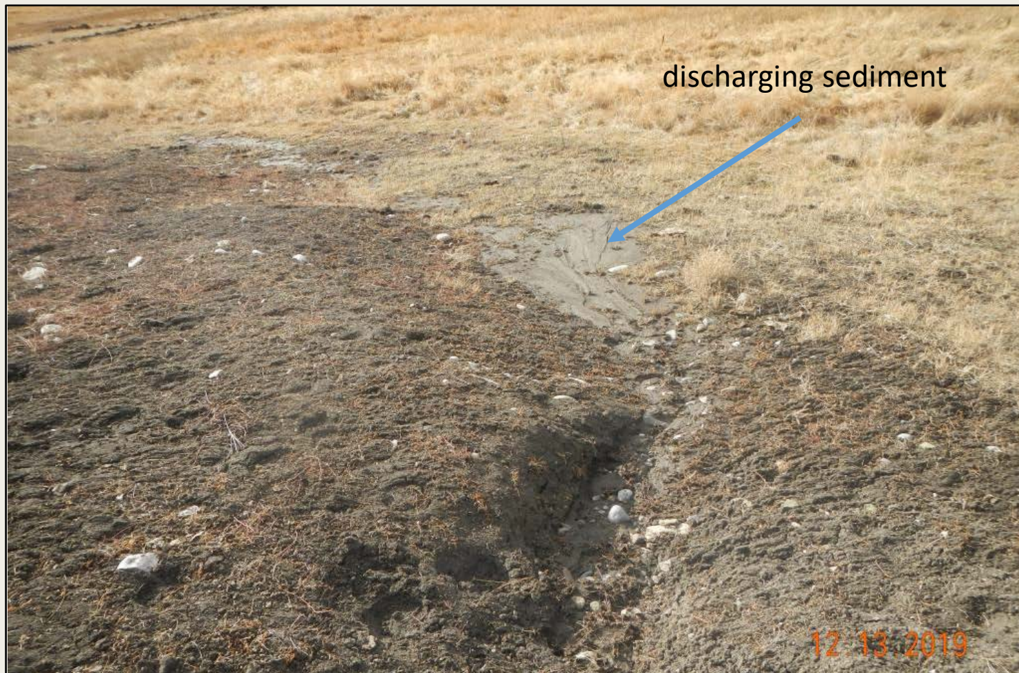
Photo 4. View of area downslope from diversion in Photo 3, where sediment is discharging off of the project area.
