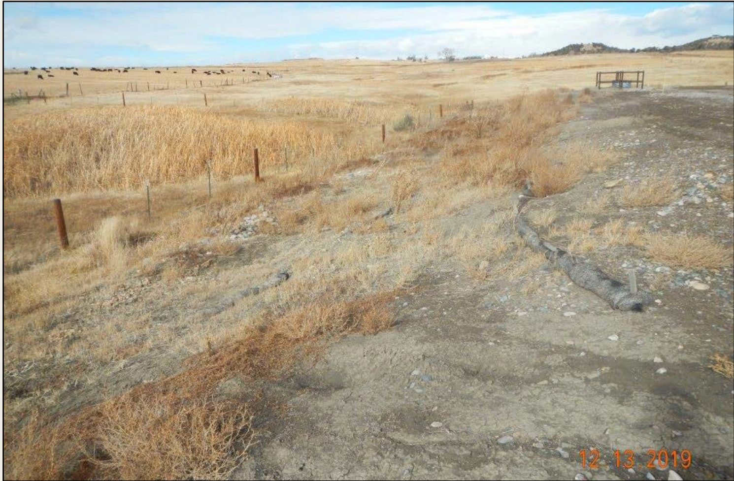
Photo 4. View of the western project area from the southwestern corner facing northward. Wattles are full of sediment and do not appear to be functioning.
