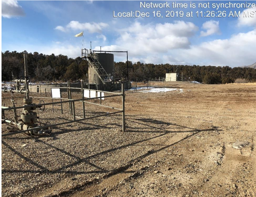
Photo #0257 photo from SW corner of location.
