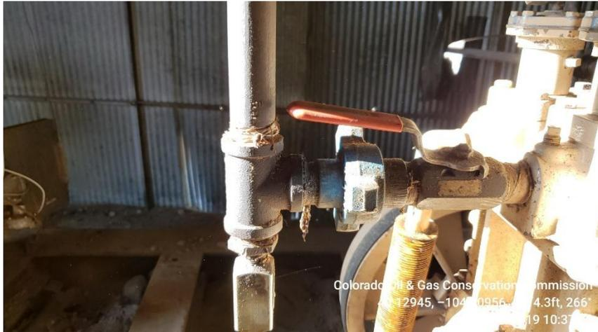
**Photo 13 hammer union appears to have been tightened**
