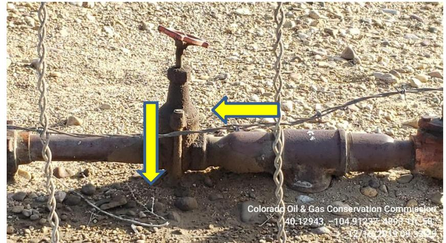
Photo 3 WH, Stained soil by valve on flow line
