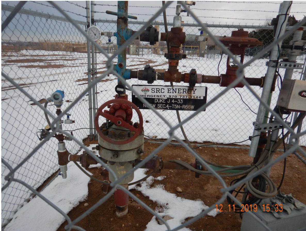
Photo 1. Photo taken from the Duke USX location. Photo illustrates only one well remains, as the other seven have been plugged and abandoned; therefore, this is a well release on an active location.
