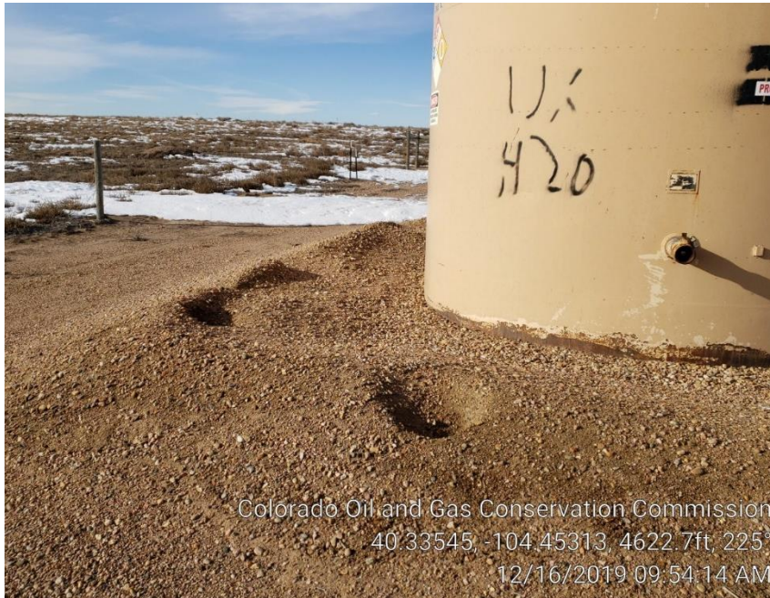
Photo #11 Inadequate berms
