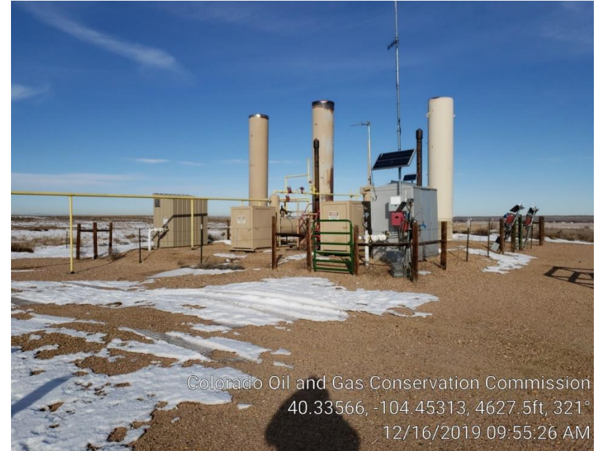
Photo #6 Separators, ECD's & Meter Runs
