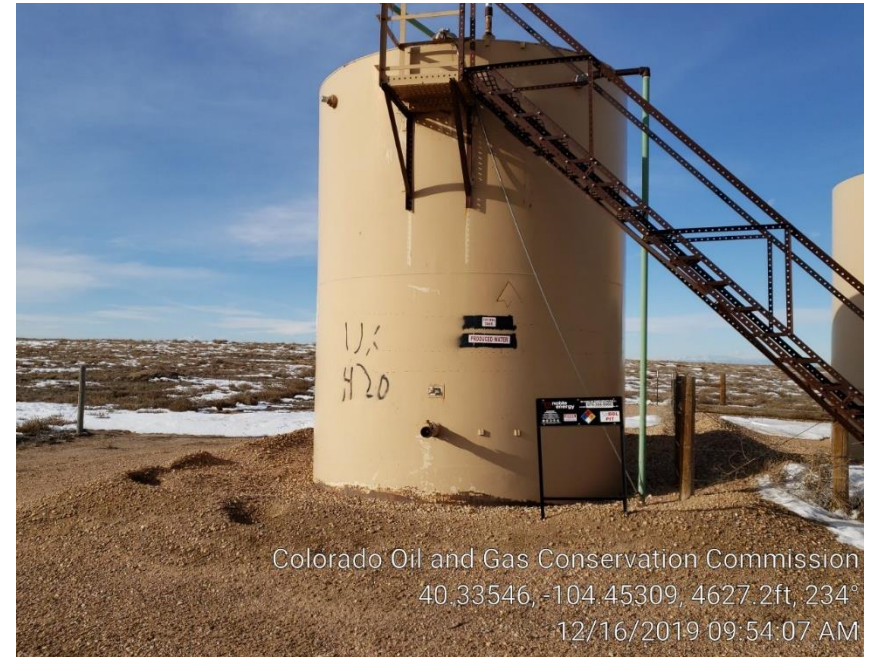
Photo #10 Water Tank/ Inadequate berms
