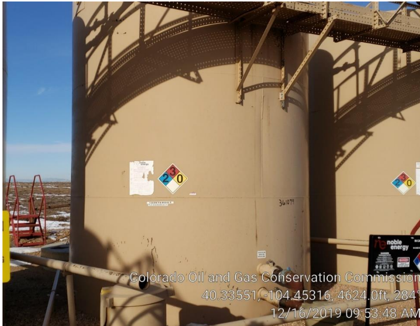
Photo #9 Missing Capacity Label
