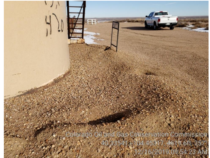
Photo #12 Inadequate berms
