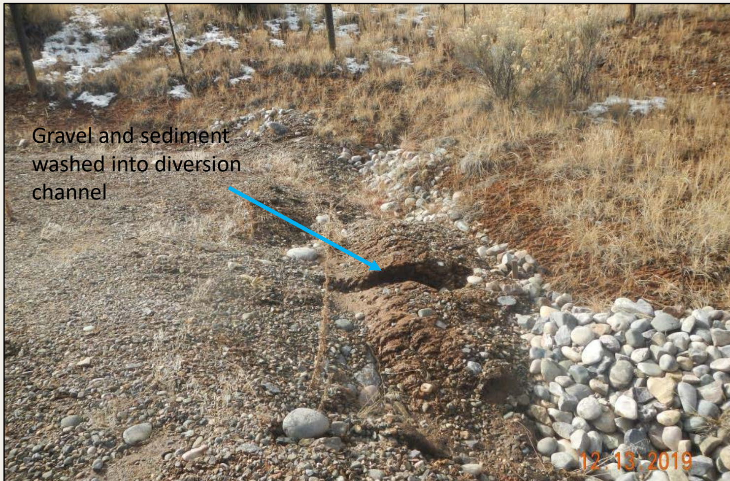
Photo 3. View of area within the northwestern well pad, where gravel and sediment washes off of the well pad into diversion channel. BMPs are full of gravel and sediment and do not appear to be the appropriate BMP for this area.
