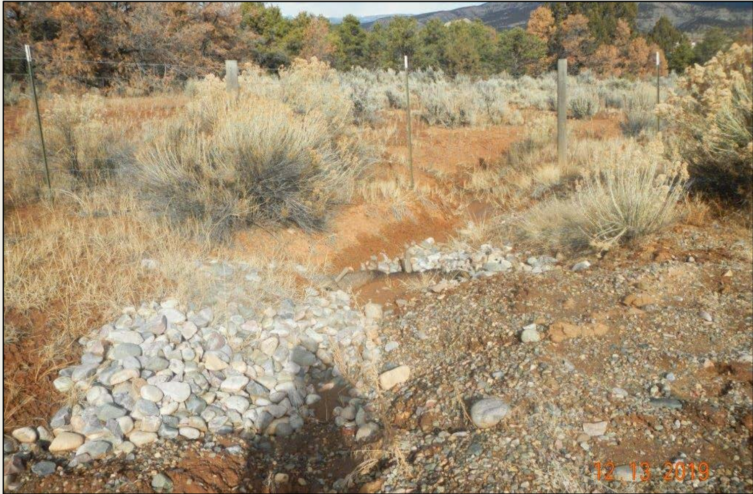
Photo 4. Another view of the northwestern project area facing northward. It appears well pad gravel and sediment washes off of the well pad into the diversion where BMPs are filling with sediment.
