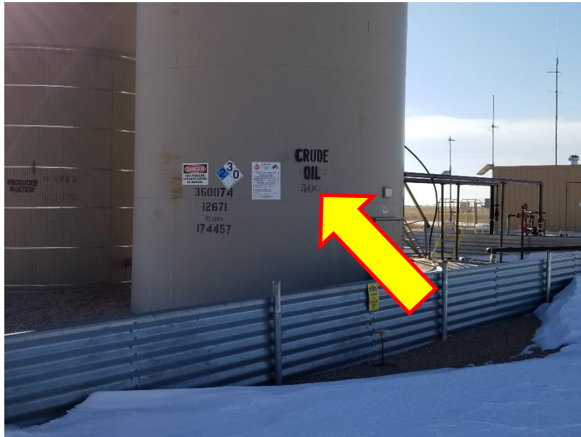
Photo 3 – Crude Oil Tank – Capacity Label has faded, no longer visible
