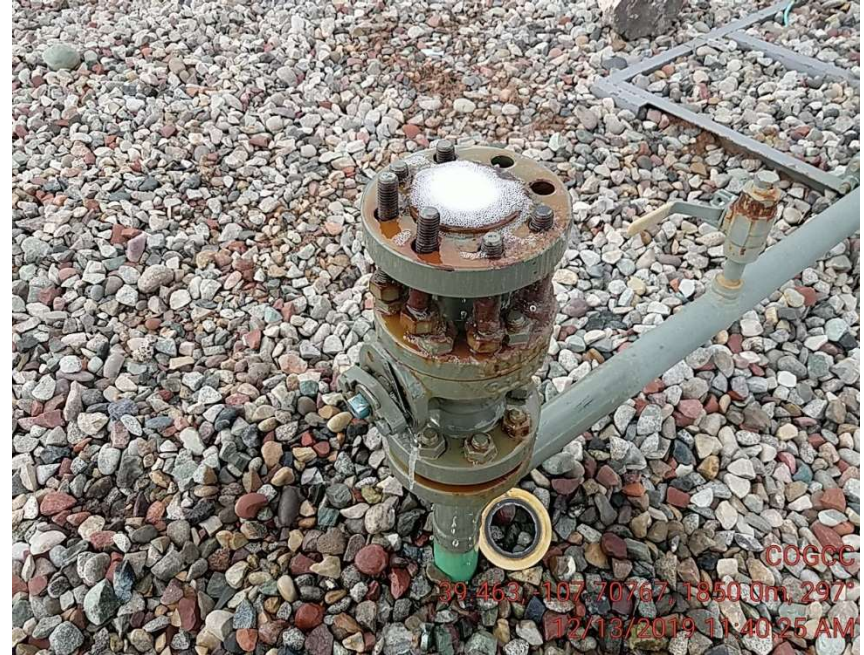
Pipe leaking
