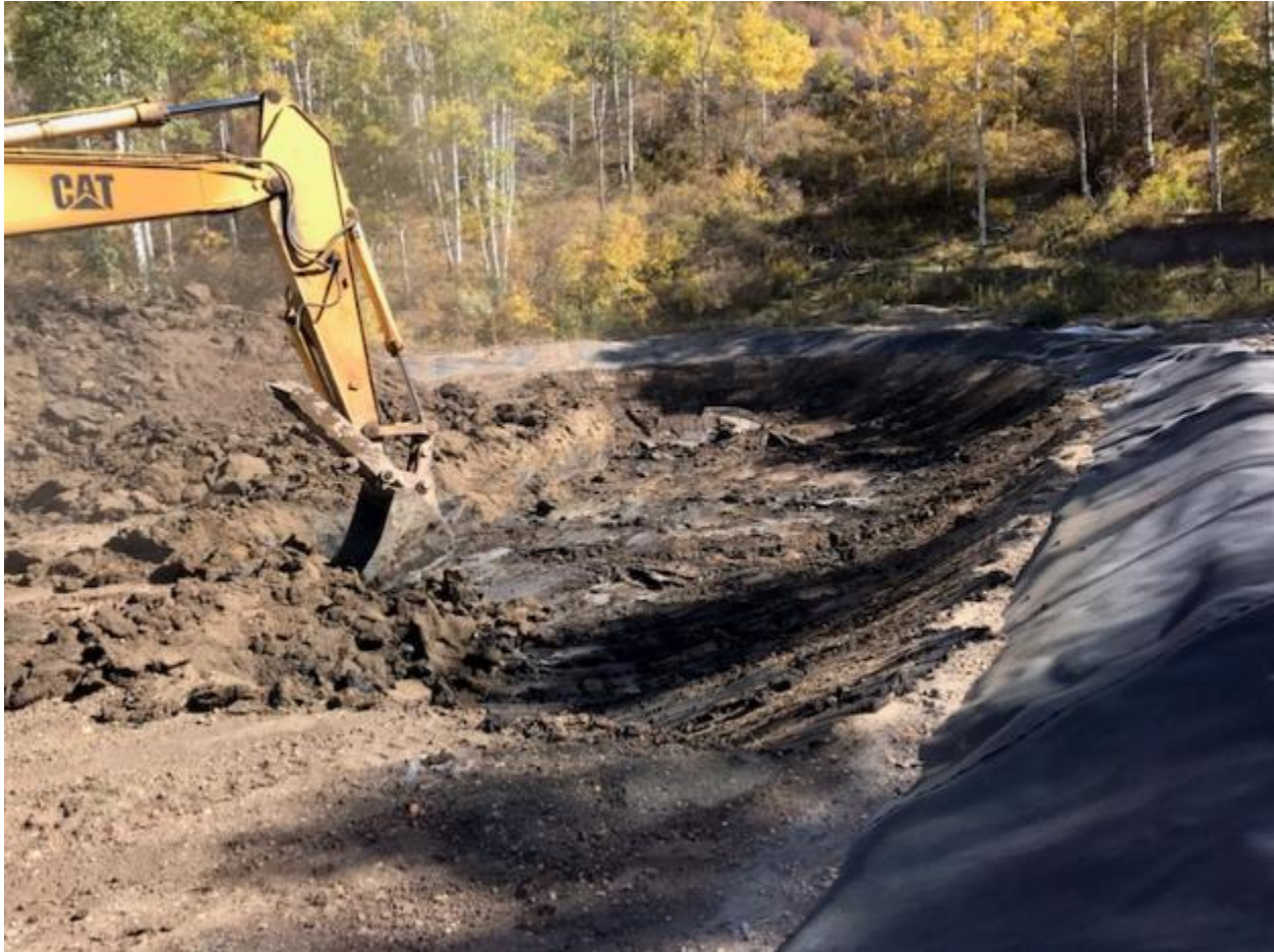
Photo 1: Landfarm Cell 1 soil removal activities.
