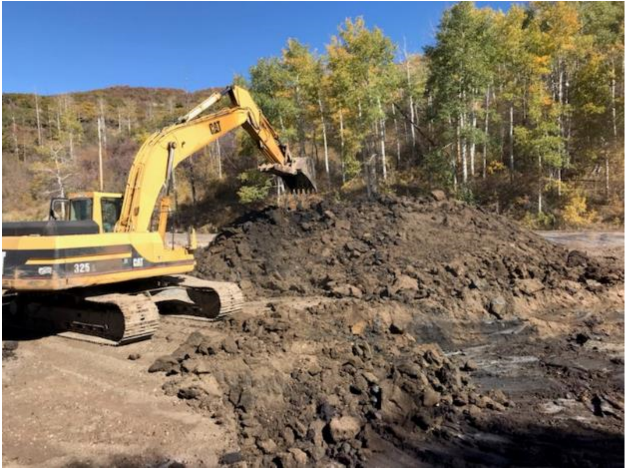
Photo 2: Stockpiling of removed soil for disposal.
