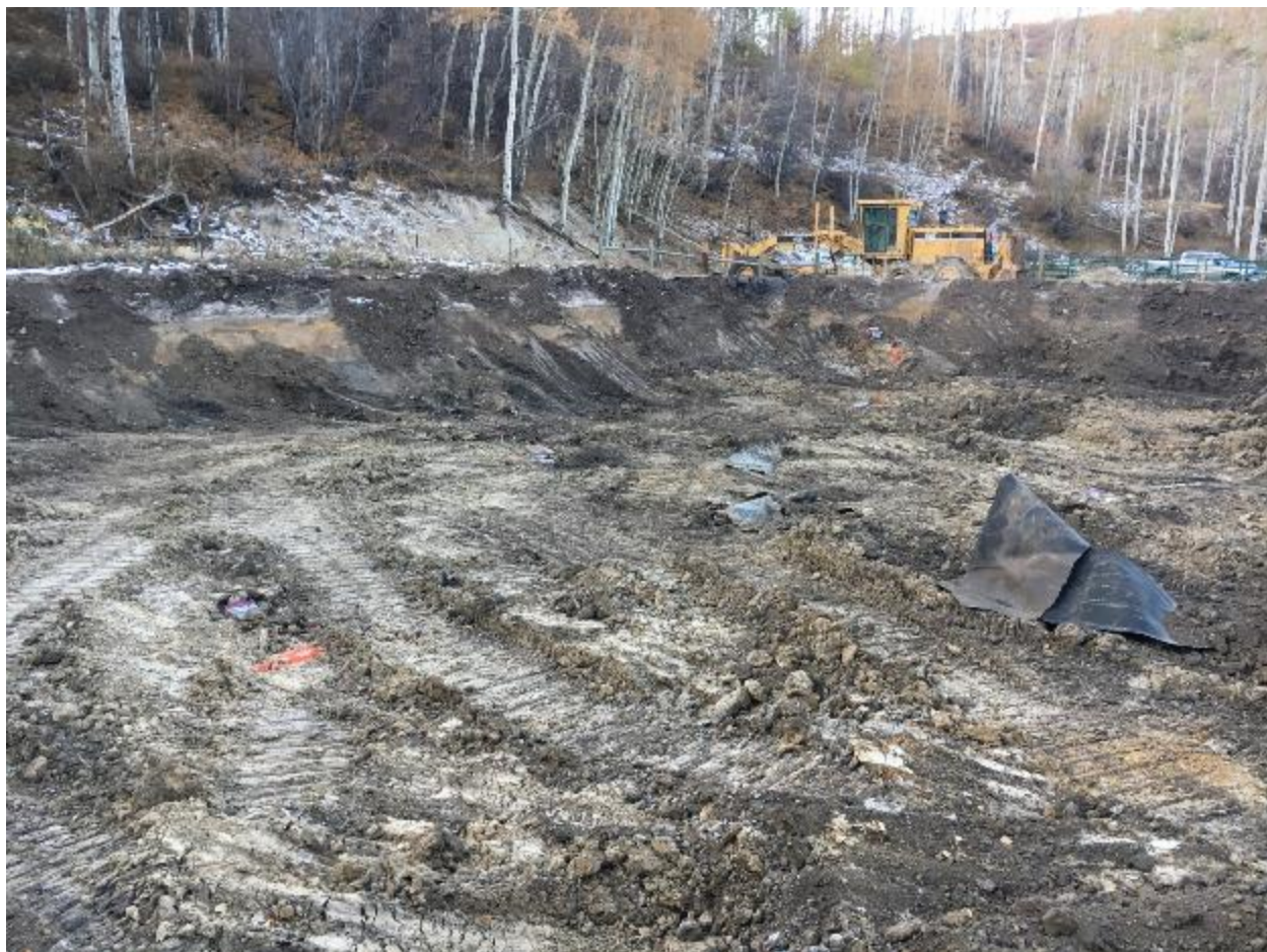
Photo 4: Base of Cell 1 area after soil and liner removal.
