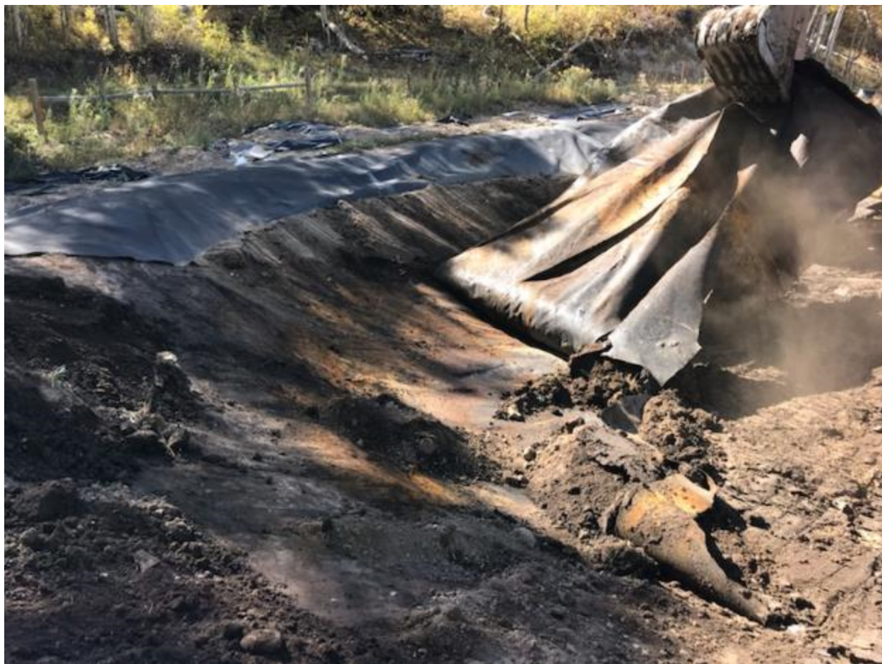
Photo 3: Removal of Cell 1 liner beneath E&P soil.
