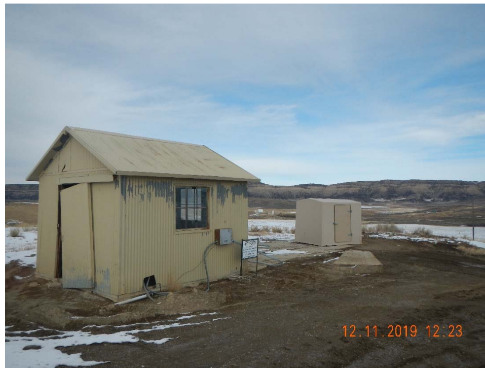
Photo 1. Overview of location taken facing north.
