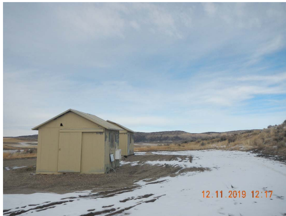
Photo 1. Overview of location taken facing north.
