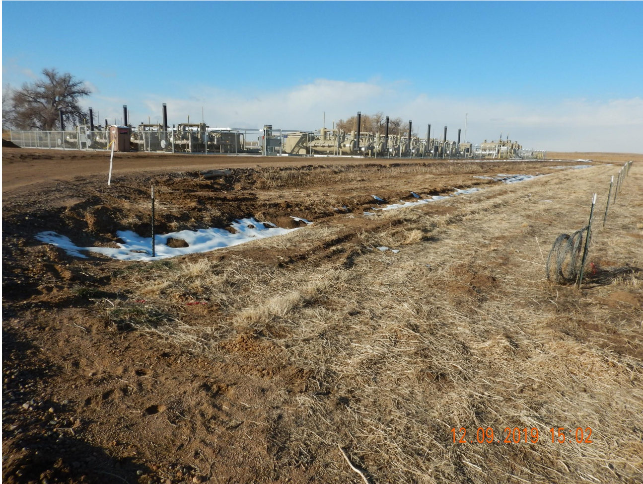
Photo 4. Photo taken from the central location, facing North. See comments under Photo 1. Also, photo illustrates perimeter ditch and berm BMP installed along the eastern location that appears to be in proper functioning condition at the time of this inspection.
