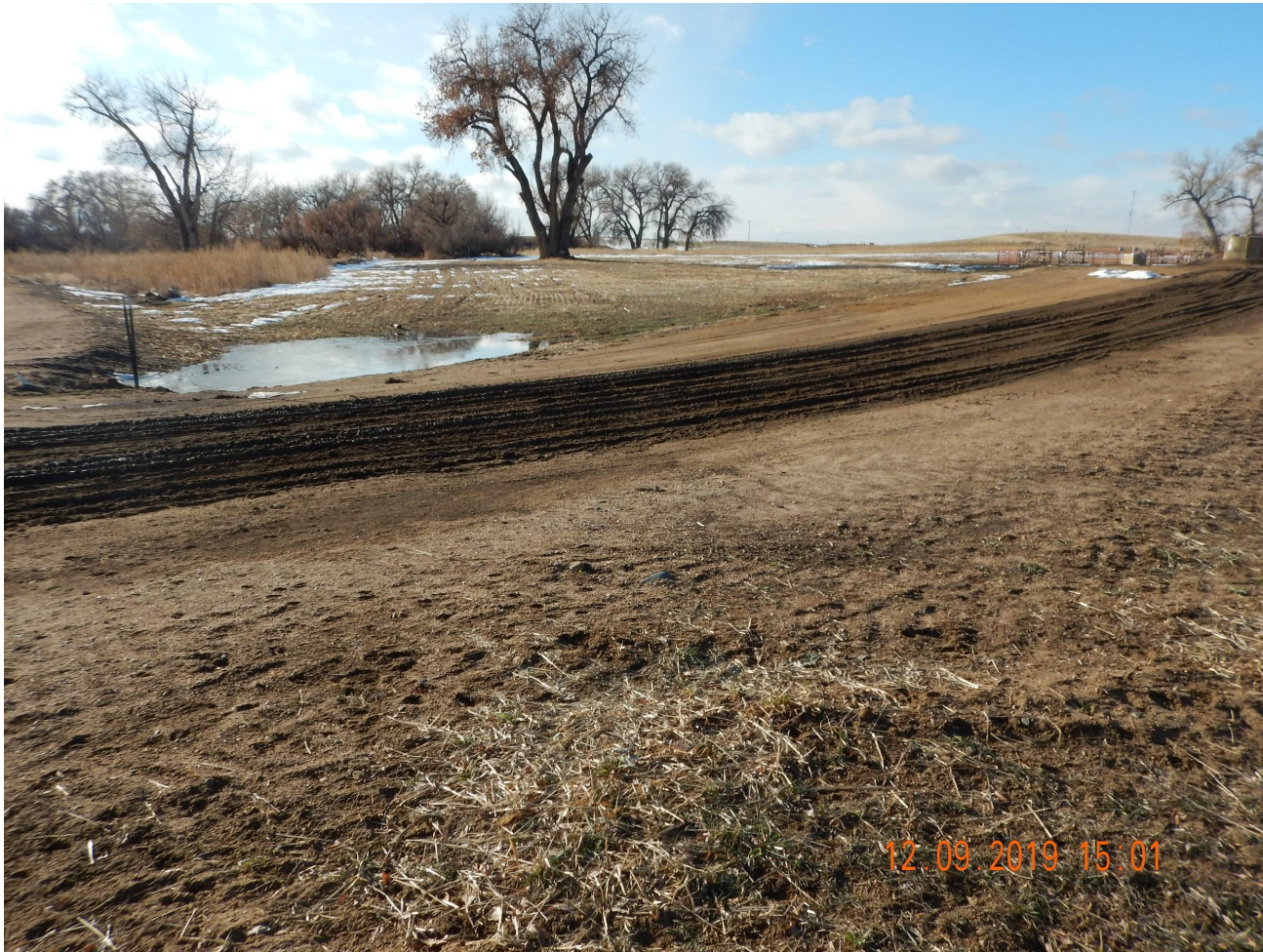
Photo 1. Photo taken from the southern location, facing West. Photo illustrates Operator has performed Interim Reclamation activities with the evidence of drill rows, straw crimped mulch and germination.
