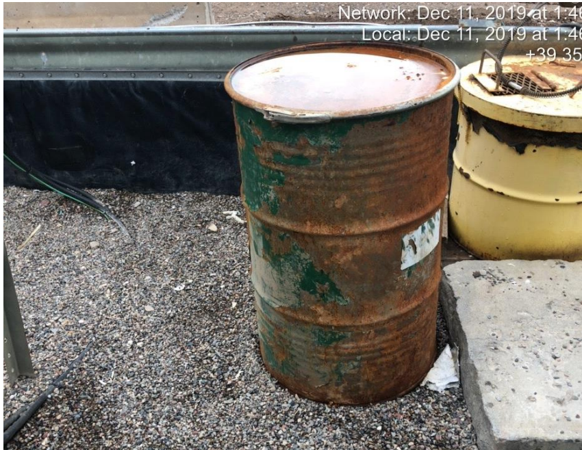
Photo #0230 Unmarked drum inside tank containment.
