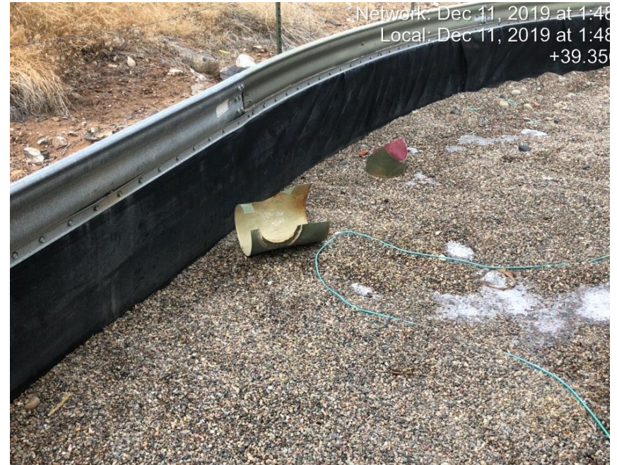
Photo #0231 trash inside containment.
