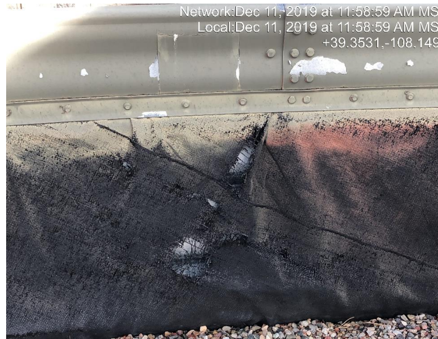
Photo #0226 Multiple holes in tank containment liner.
