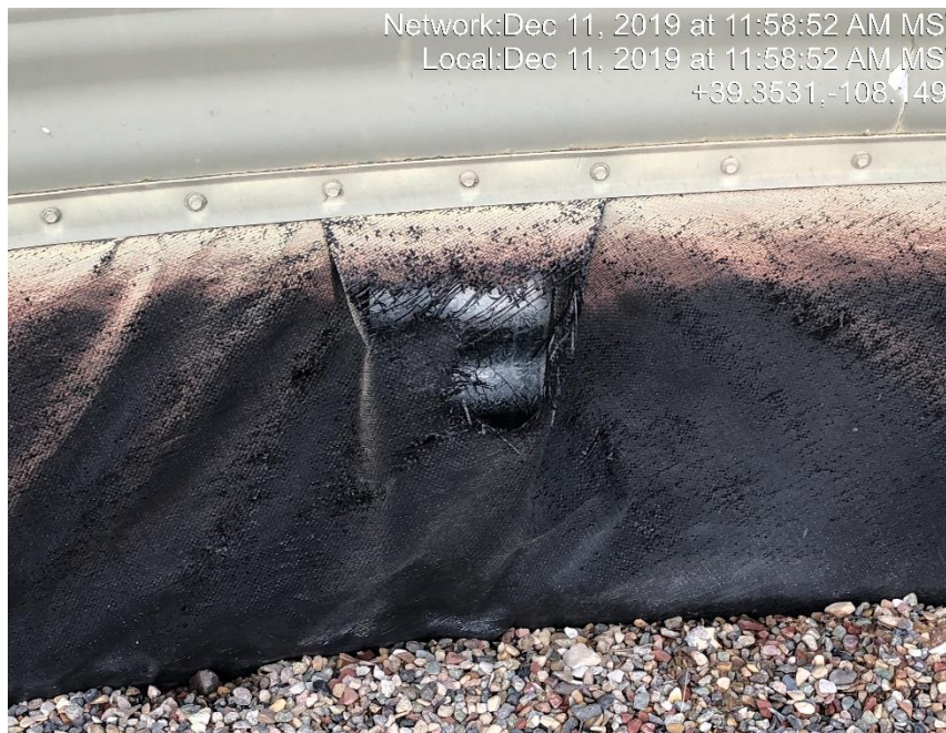
Photo #0225 Multiple holes in tank containment liner.
