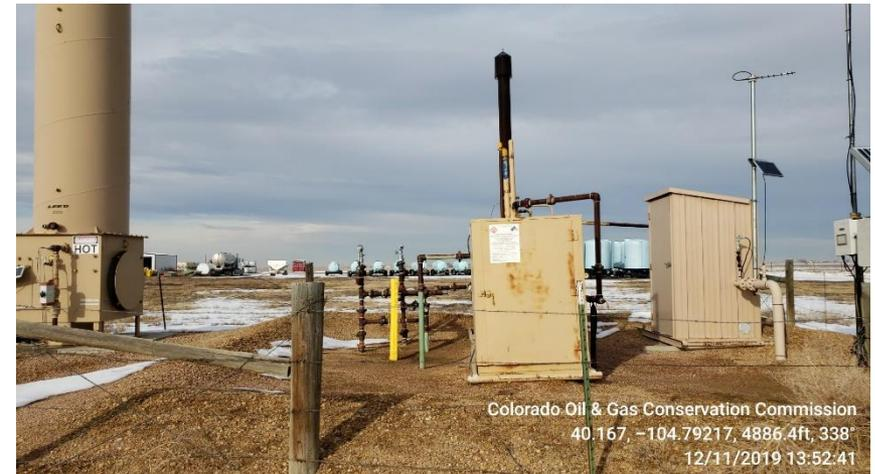
**Photo 3 Horz. Heated Sep., as meter run**
