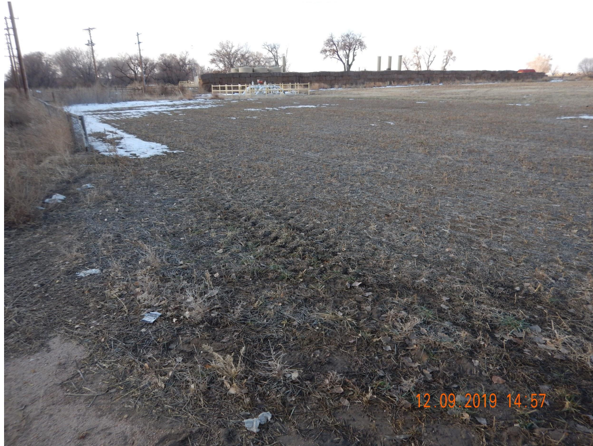
Photo 1. Photo taken from the tank battery location, facing West. Photo illustrates the Operator has performed additional reclamation activities in response to the previous corrective action inspection with the evidence of drill rows, straw crimped mulch and some germination.
