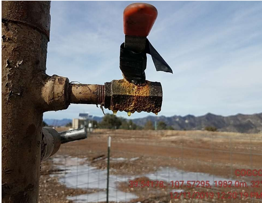
LEAKING FITTINGS PUMPER FIXED WHILE ONSITE
