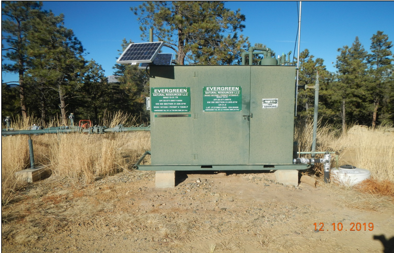
Photo 1. Well sign is installed at location.
