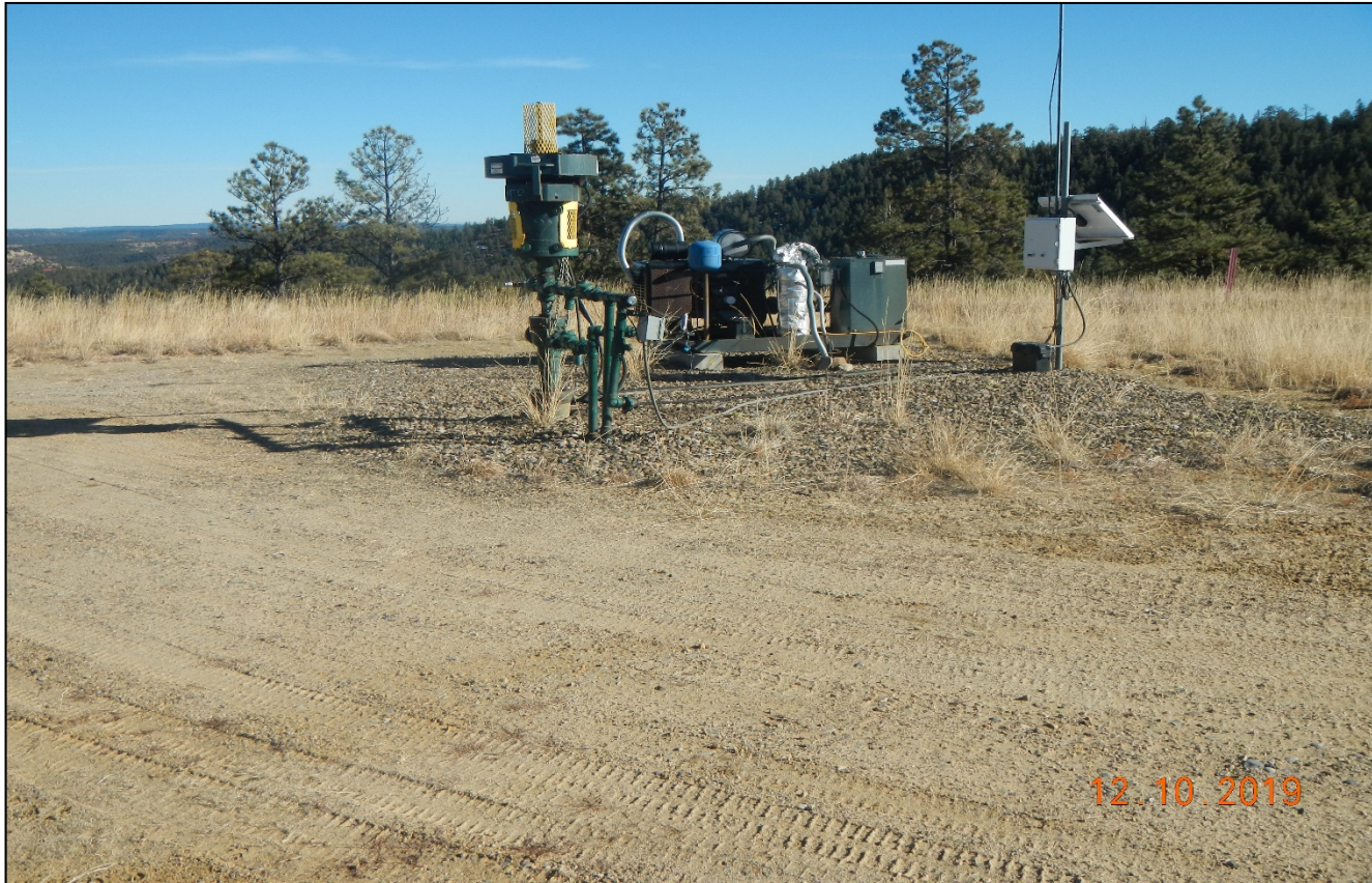
Photo 3. Facing toward the well.
