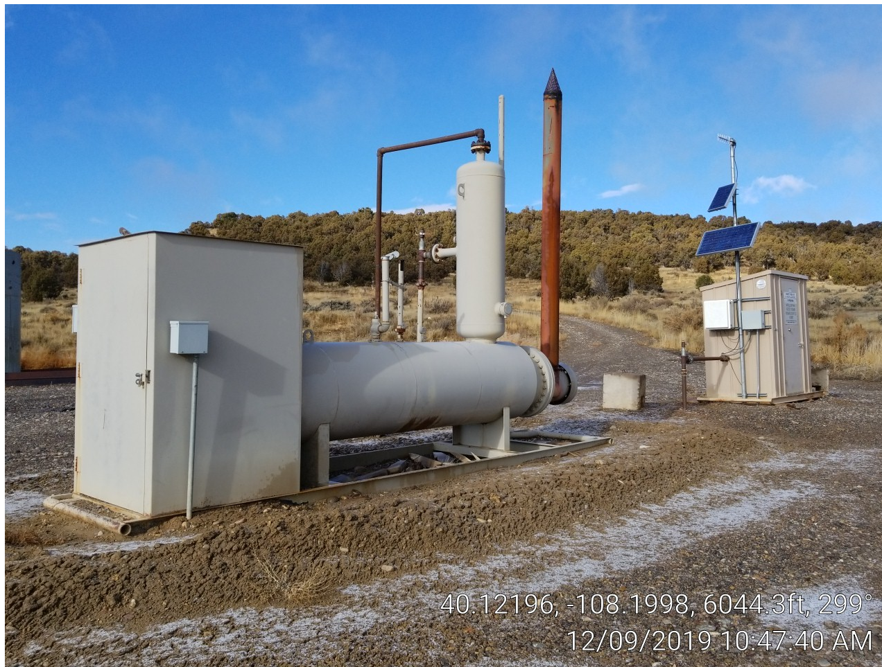
Photo 3. Separator & gas meter building.
