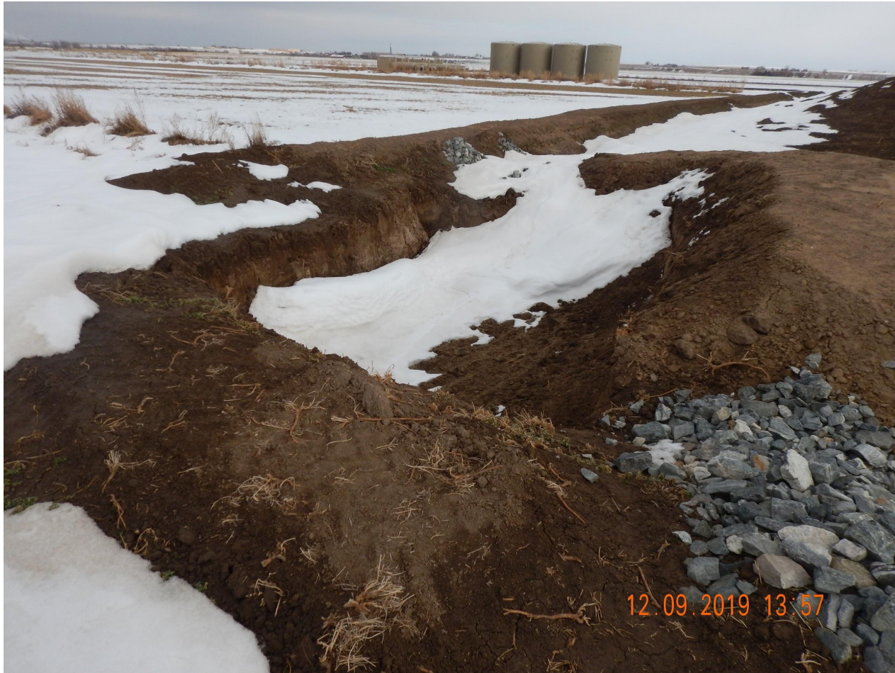
Photo 4. Photo taken from the western location, facing East. Photo illustrates Operator has installed a sediment trap in conjunction with the ditch and berm BMPs. Operator has not constructed the sediment trap with good engineering practices, as the side slopes should not be vertical (1:1) but rather 2:1 slope or flatter.
