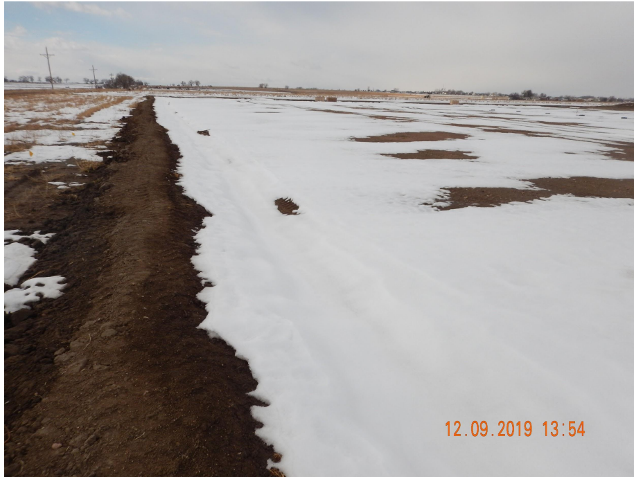
Photo 2. Photo taken from the southern perimeter of location, facing West. Photo illustrates a ditch and berm BMP.
