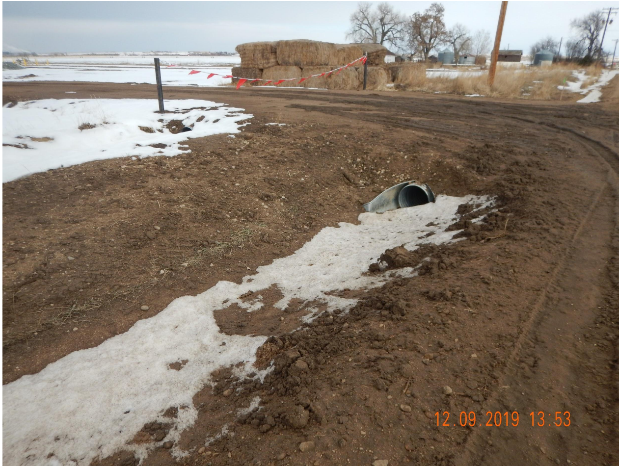
Photo 1. Photo taken from the entrance of location, facing East. Photo illustrates Operator has installed culverts, one of which is in conjunction with the roadside ditch.
