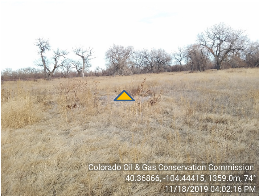
Photo #1 DOW 23-28 (05-123-20593) Wellsite Plugged & Abandoned | PA ~ 15 yds. Appears to be cut & capped Reclamation progressing prior insp.
