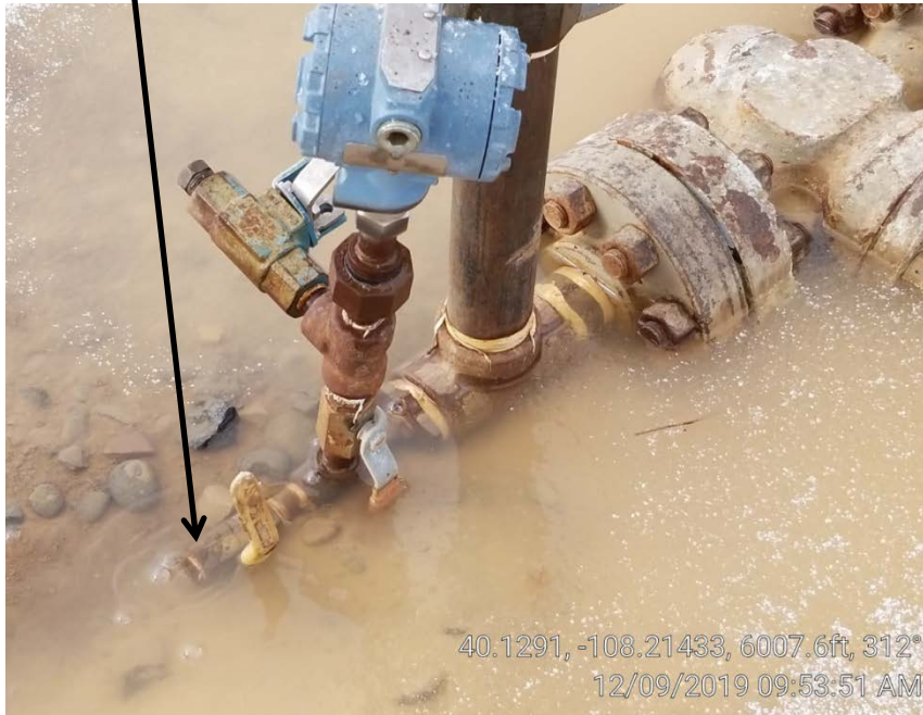
Photo 6. Leaking valve.
