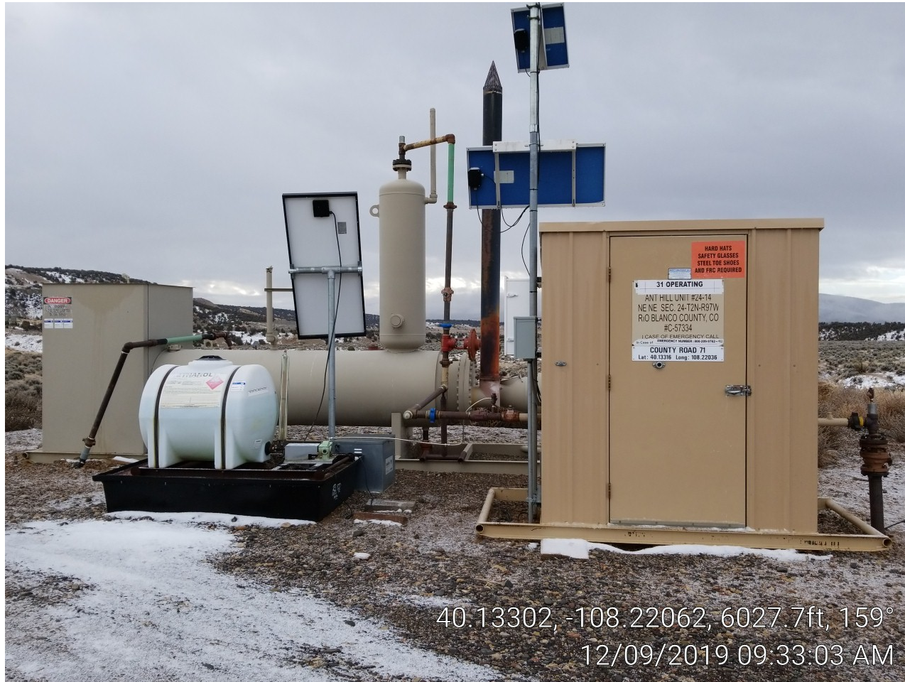
Photo 2. Meter building & separator.
