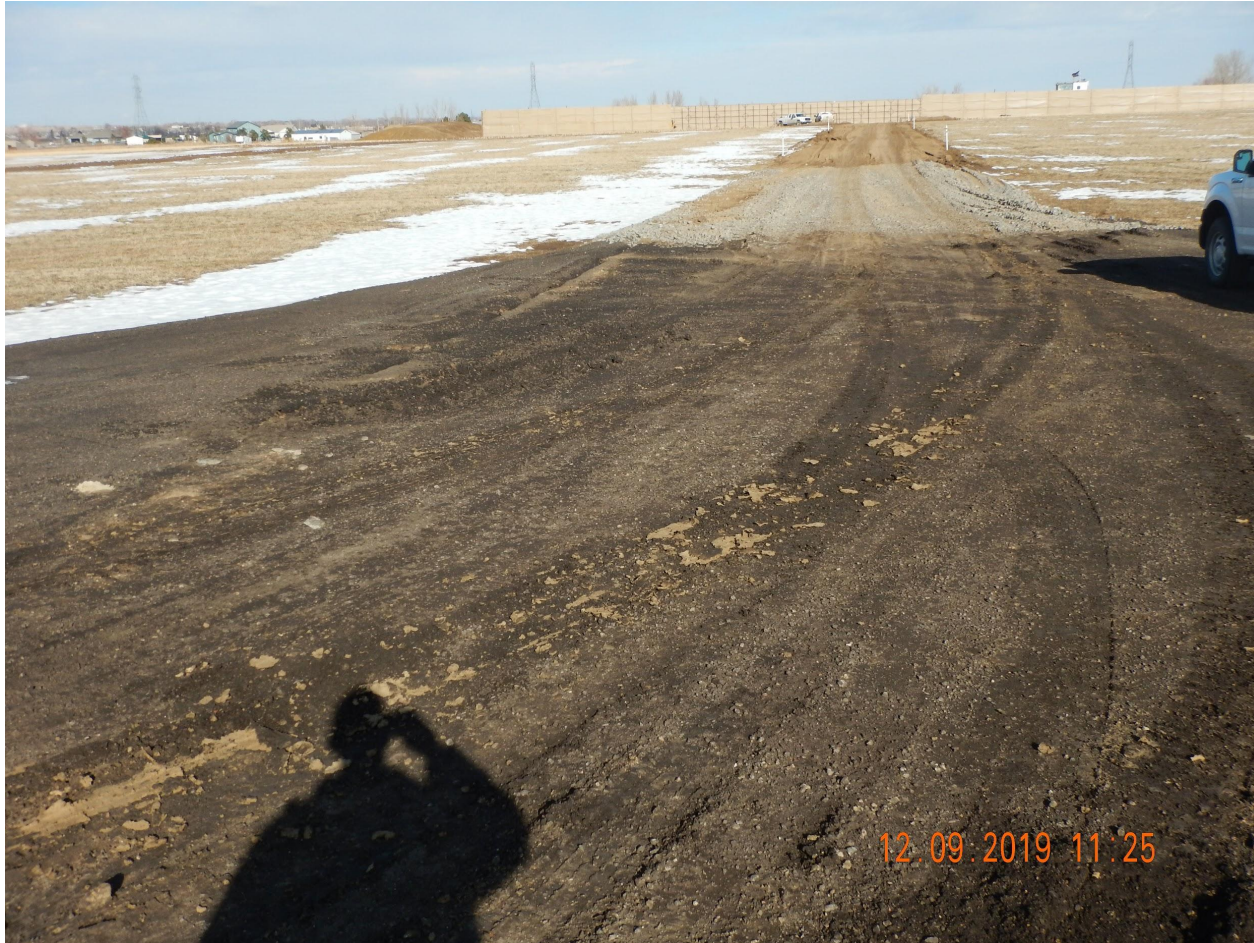
Photo 2. Photo taken from the entrance of the location, facing North. The current vehicle tracking device BMPs are not adequate to be in compliance with Rule 1002.f.(2)F.
