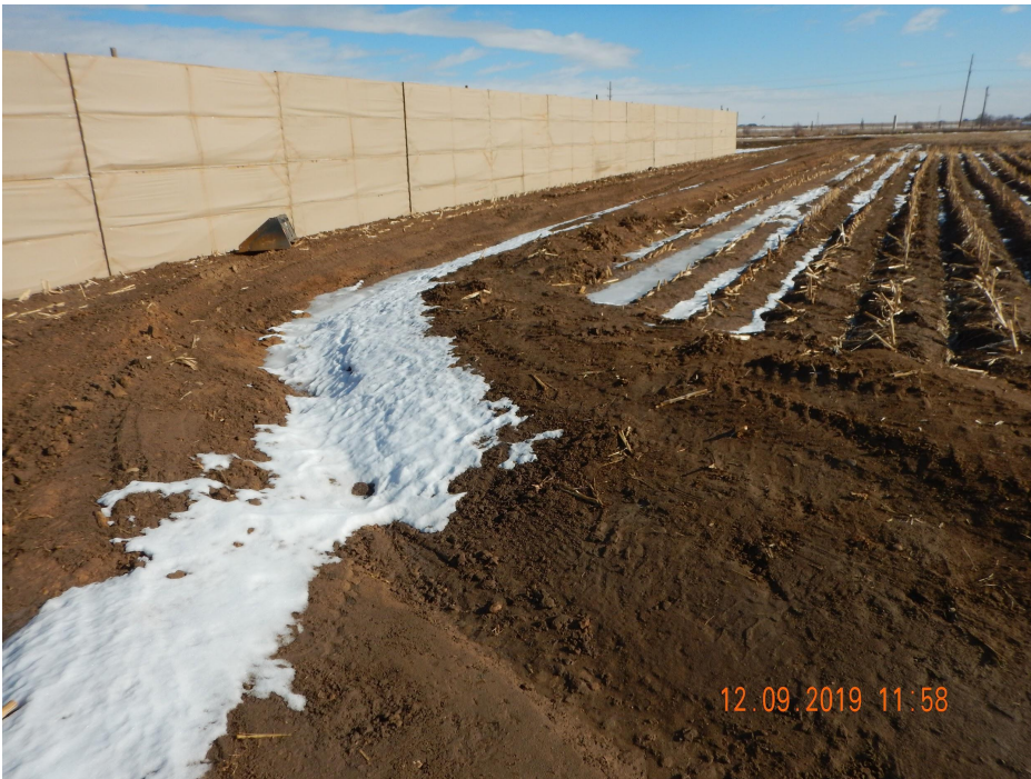
Photo 4. Photo taken from the southern location, facing East. Photo illustrates a ditch and berm BMP that has been installed around the entire perimeter of location.
