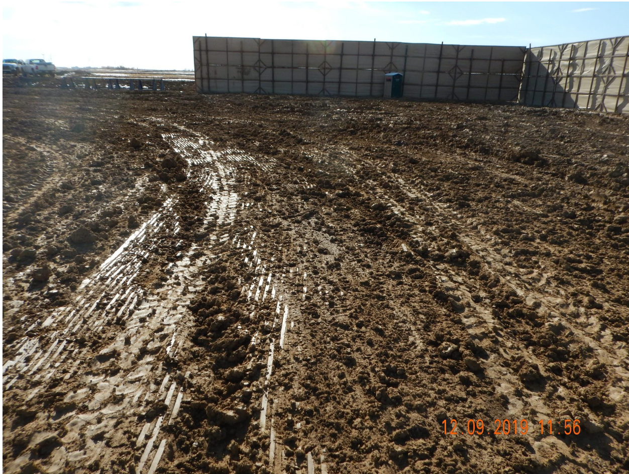
Photo 3. Photo taken from the location, facing South. Photo illustrates the current muddy conditions. Operator has not plated the location making it susceptible to muddy conditions and continued track out.
