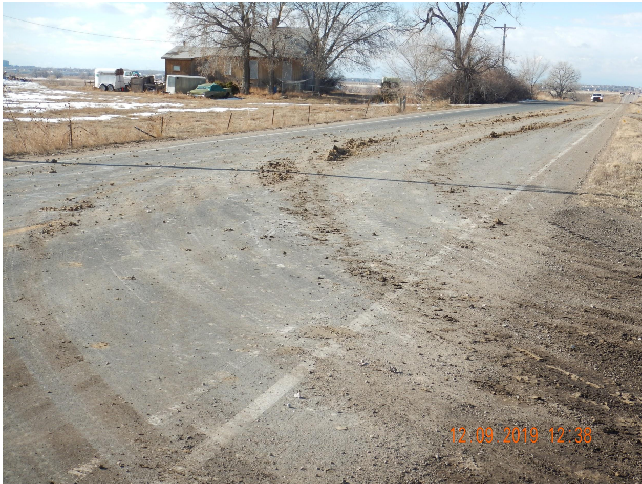
Photo 1. Photo taken from the entrance of the location off CR 2, facing West. Photo illustrates sediment track out onto CR 2. The current vehicle tracking device BMPs are not adequate to be in compliance with Rule 1002.f.(2)F.
