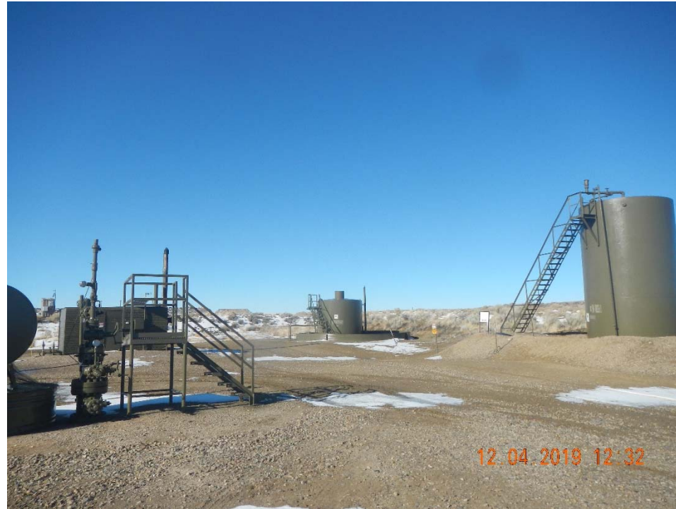
Photo 1. Overview of location taken facing north.
