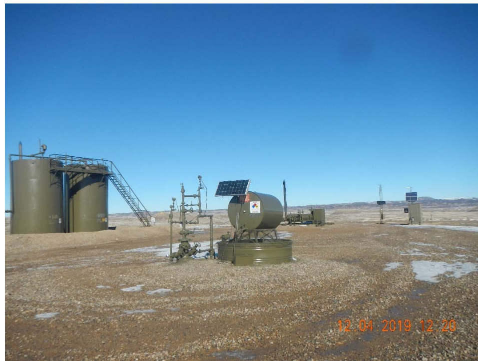
Photo 1. Overview of location taken facing north.
