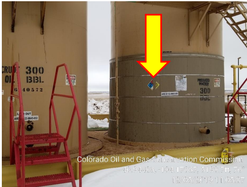
Photo 3 – NFPA Label has peeled off
