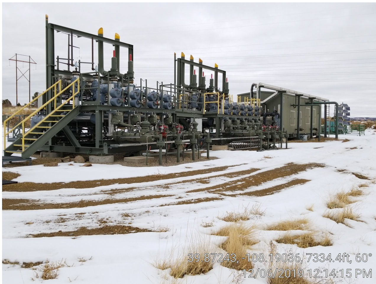
Photo 4. Well manifold & separator.
