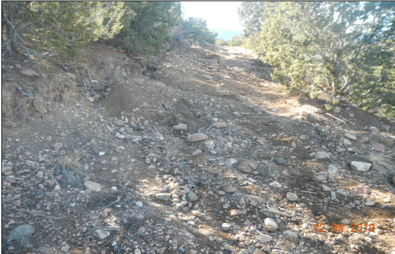
Photo 8. Facing southwest along the access road between the Hassler 24 and Drapper 4 well site. It appears soil material has been pushed over the road however, the recontouring and reclamation have not been completed.
