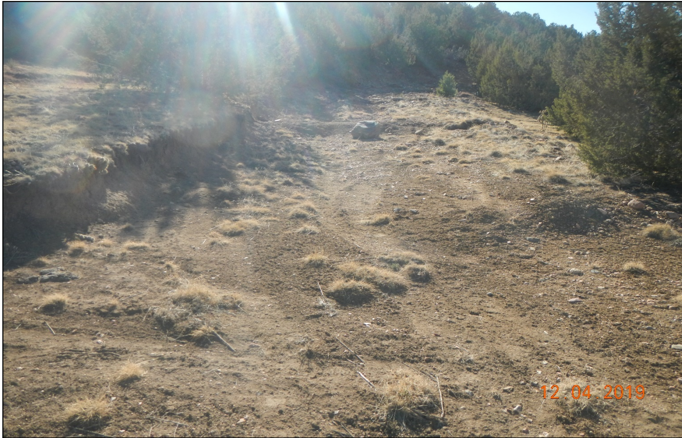
Photo 9. The old access road begins near the Drapper 4 well site. The access road has not been recontoured and reclaimed.
