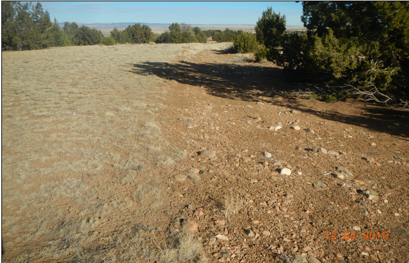
Photo 1. Facing north at the access road from CR 103. Access road has not been reclaimed and is bare of vegetation. Vegetation growth at left portion of the photo is undisturbed reference area.
