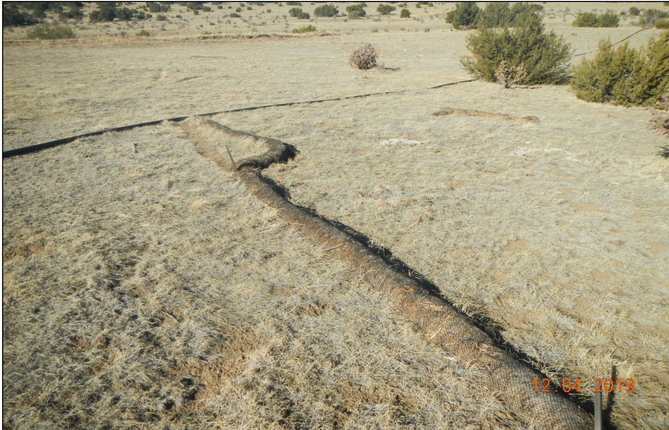
Photo 5. There are degraded and displace wattles at the north side of the location.
