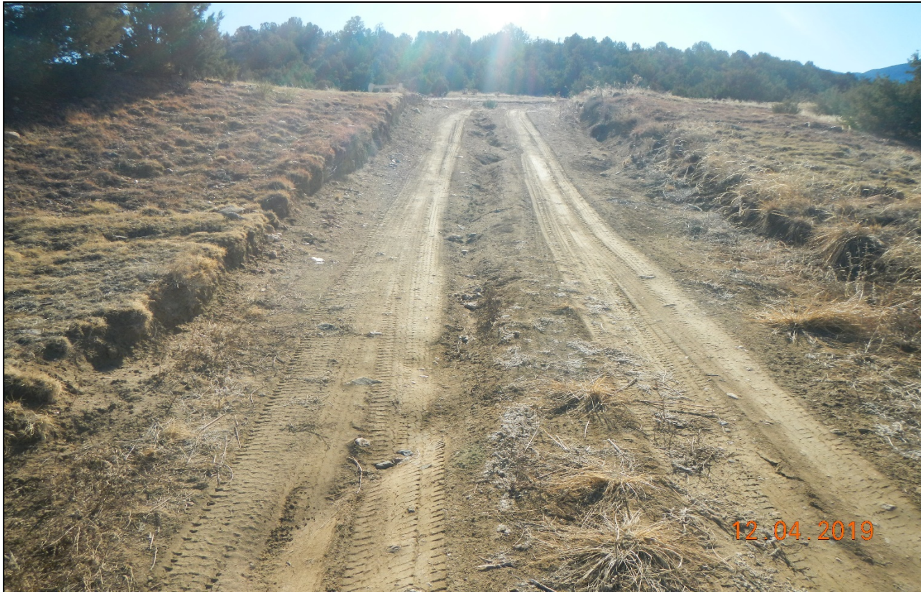
Photo 3. Facing south along the access road. There is vehicle rutting and erosion along the access road toward the location.
