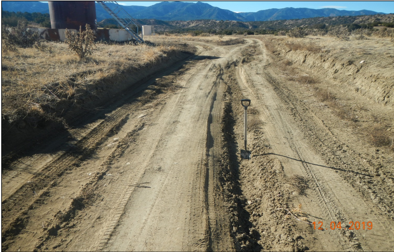
Photo 1. Facing southwest along the access road. There is vehicle rutting and erosion along the access road toward the location.
