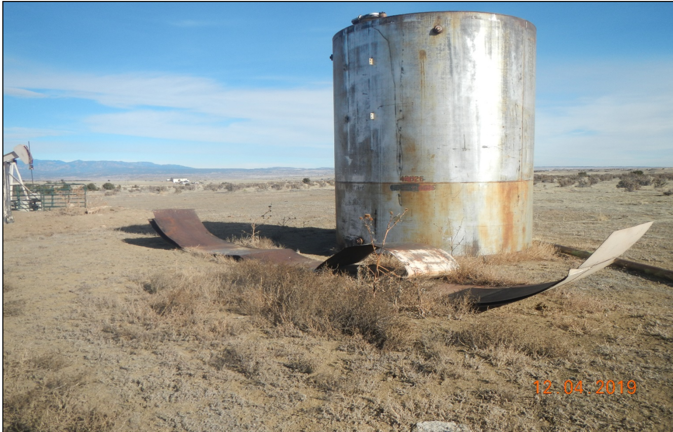
Photo 2. There is an unused tank, pipe, and metal containment stored at the location. Unused equipment must be removed.
