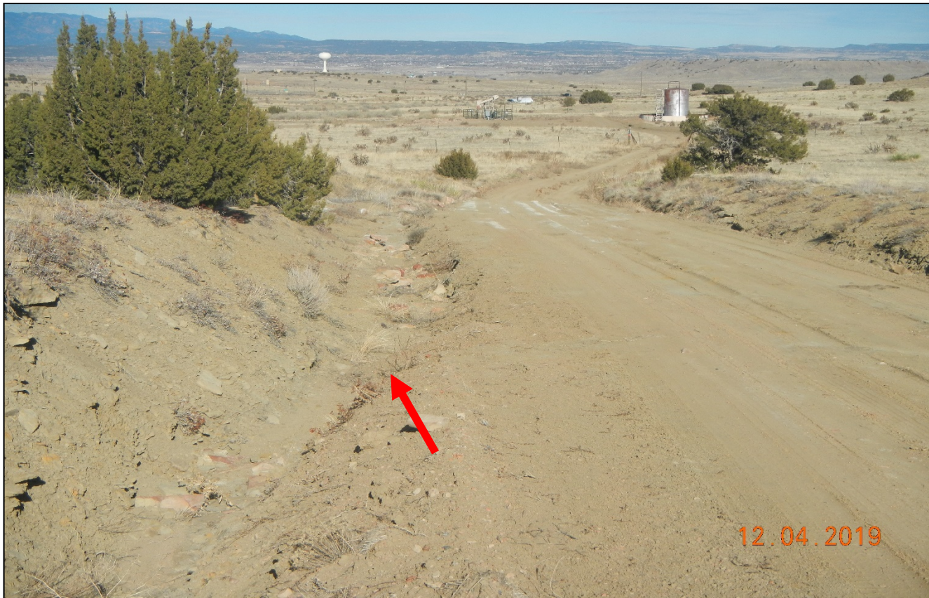
Photo 4. There is erosion occurring along the road toward the location. No BMP's are installed to prevent erosion.
