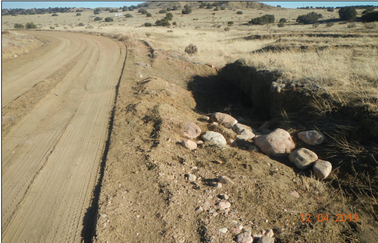
Photo 1. The erosion along the access road has not been repaired and stabilized. It appears rocks were placed at the erosion channel but are inadequate and not installed per good engineering practice. (Lat/Long:38.33276,-105.11330)
