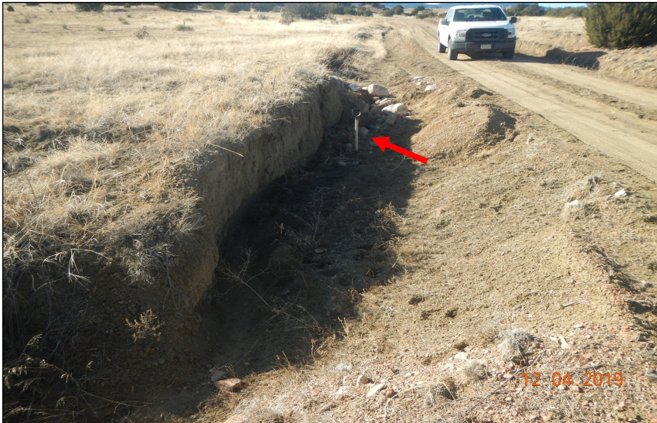
Photo 2. View of the erosion channel along the access road. Arrow points to 3.5 ft. shovel placed in the channel to show depth and size.
