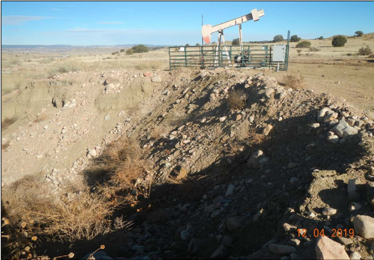
Photo 6. It appears additional material has been placed in the embankment near the wellhead. This material is loose and not stabilized.
