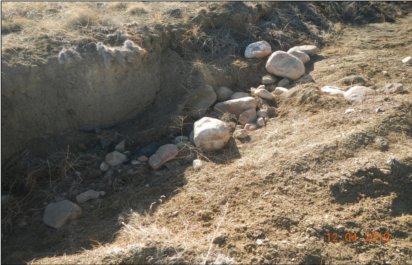
Photo 3. View of rocks placed in channel which is not properly installed and is not an effective stormwater control.
