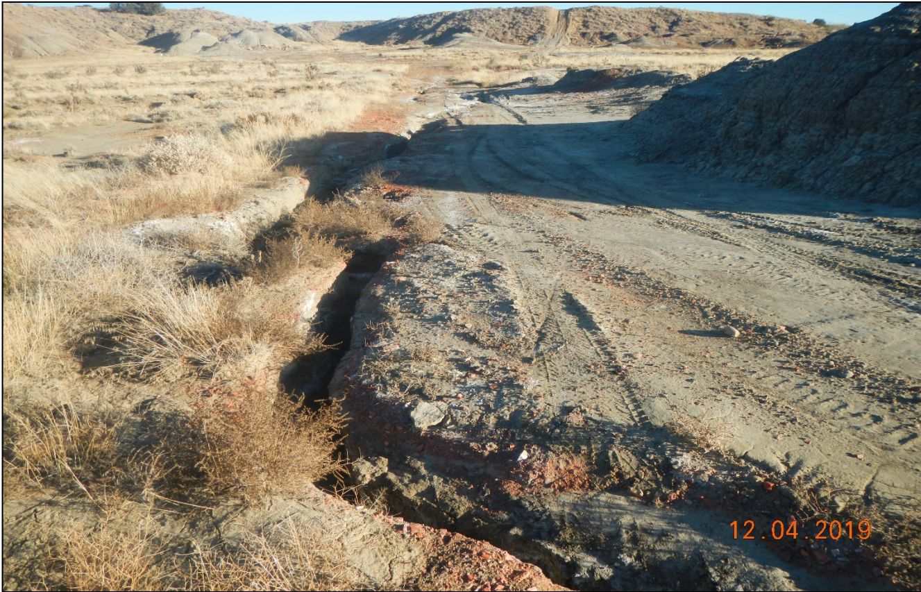
Photo 2. Facing back toward the east. There is a deep erosion channel that has degraded the main access road that must be repaired.
