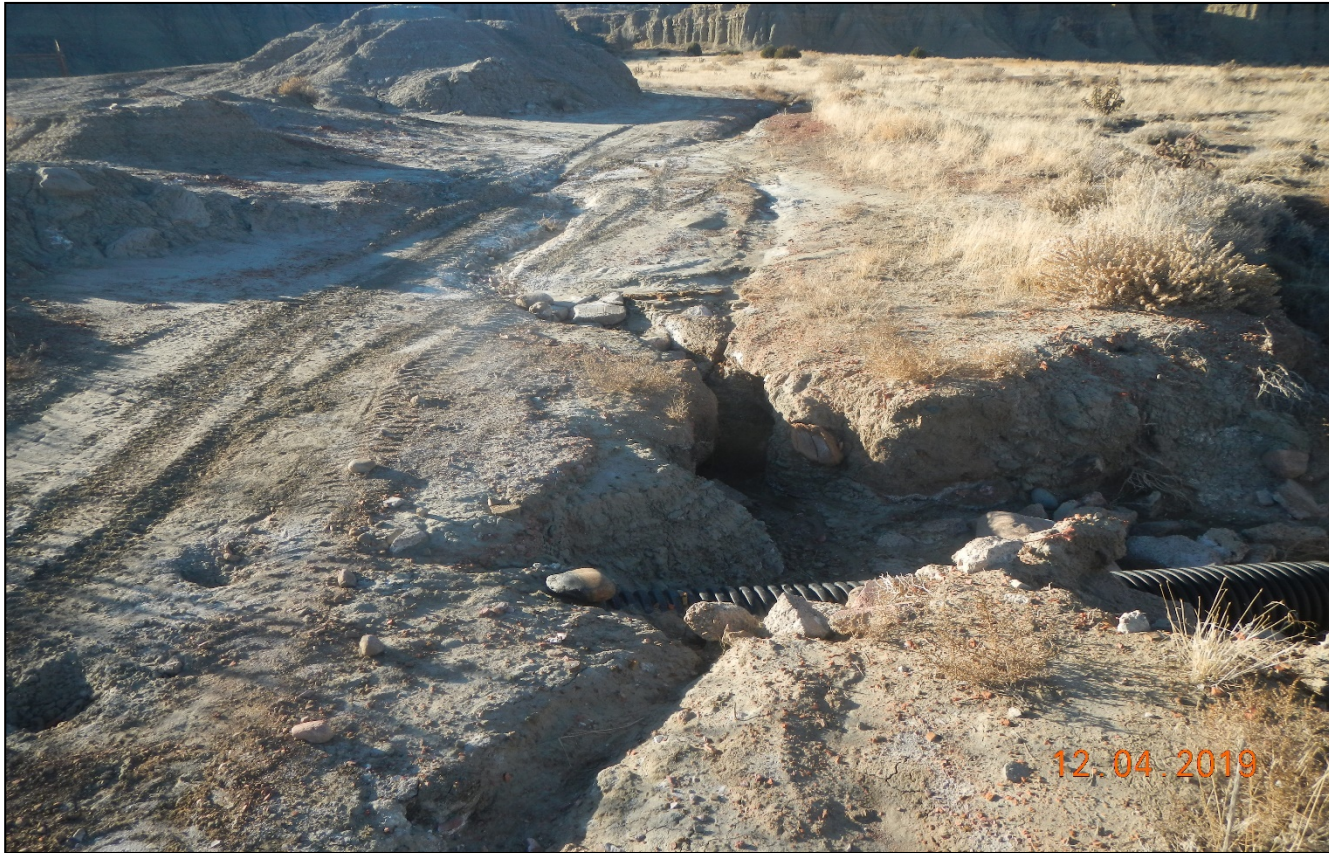
Photo 1. Facing west along the access road. There are erosion issues that must be repaired.
