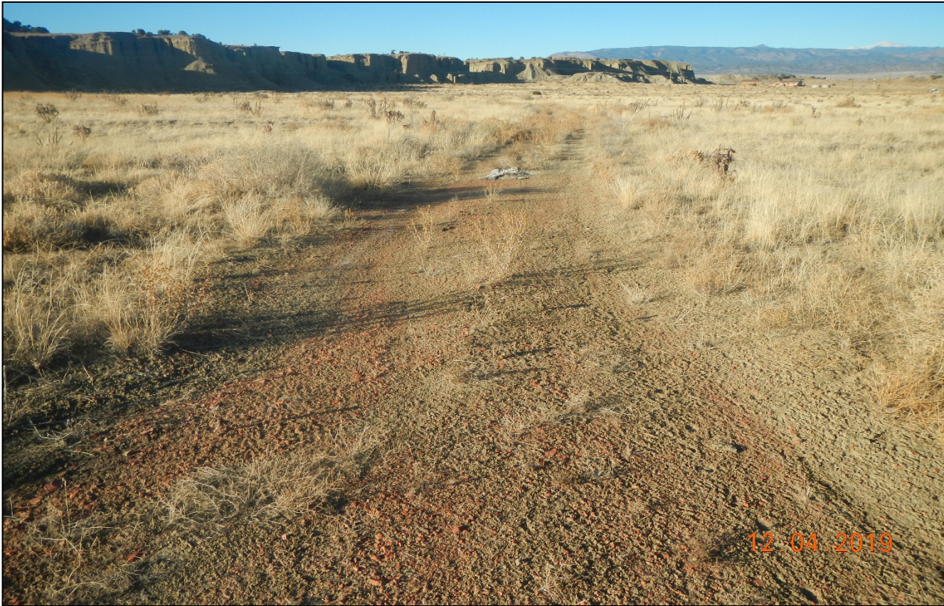
Photo 3. Facing northwest toward the access road. This portion of the access road which goes to the location must be reclaimed.
