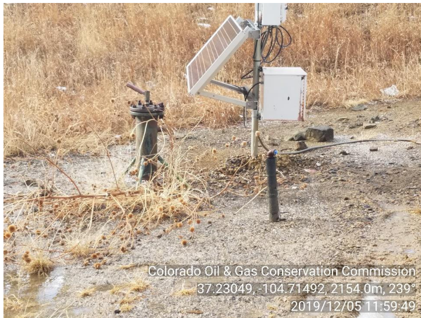
PHOTO 3: UNUSED EQUIPMENT( 1 FUEL CAN SEPARATOR AND ONE 1" UNUSED RISER). REMOVE UNUSED EQUIPMENT IN ACCORDANCE WITH NTO AND RULE 603.f. CA DATE 02-05- 20
