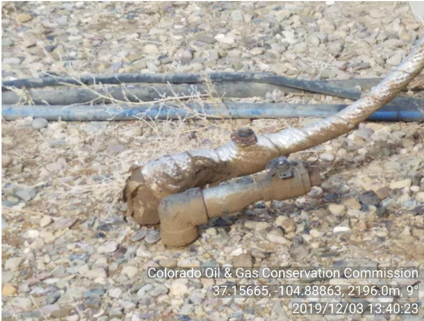
PHOTO 3: UNUSED UNMARKED RISER NEAR ENGINE SKID. REMOVE UNUSED RISER IN ACCORDANCE WITH NTO AND RULE 603.f. CA DATE 2-3-20
