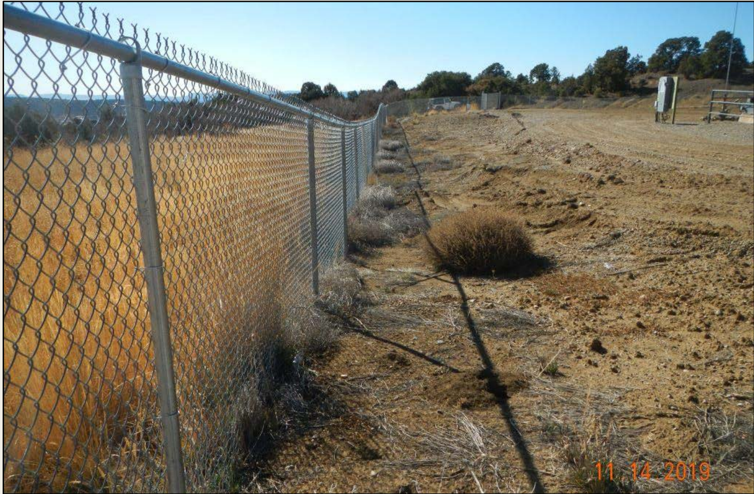
Photo 2. View of the eastern project area, within the fenced working area. Stormwater flows from the well pad are eroding the area off of the road surface, which is not vegetated with desirable vegetation.
