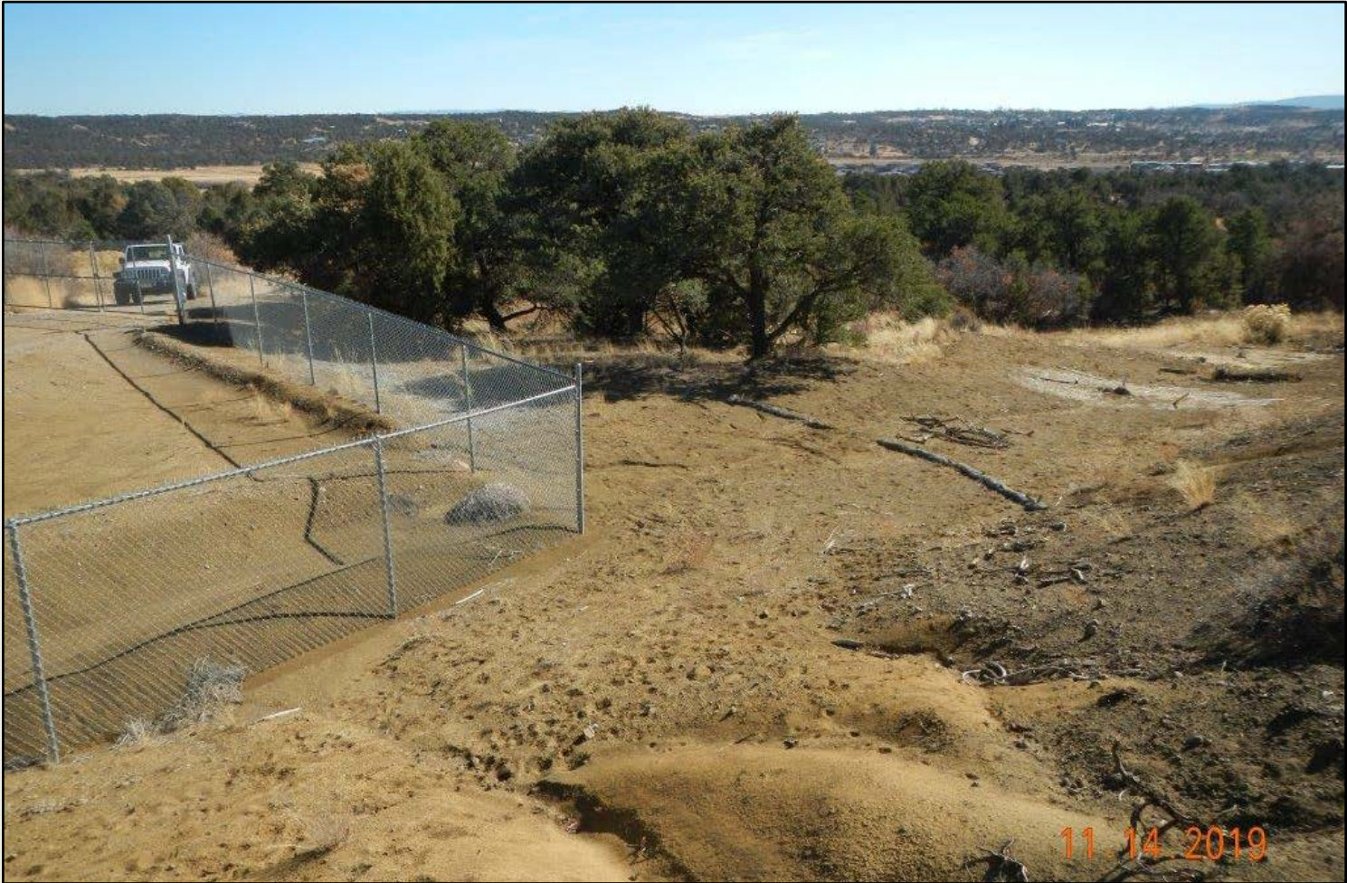
Photo 5. View of erosion and sedimentation in the southwestern project area, facing down-slope from the western cut-slope.
