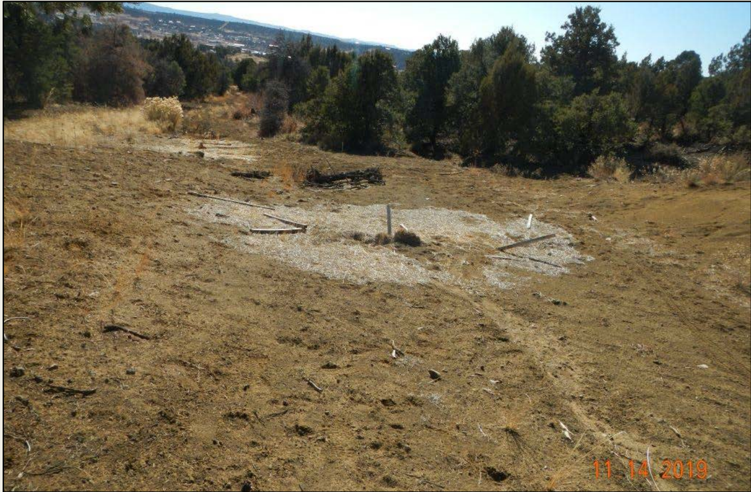
Photo 4. Another view of sedimentation and failed BMPs in the southwestern project area. Area needs stabilization measures and revegetation.
