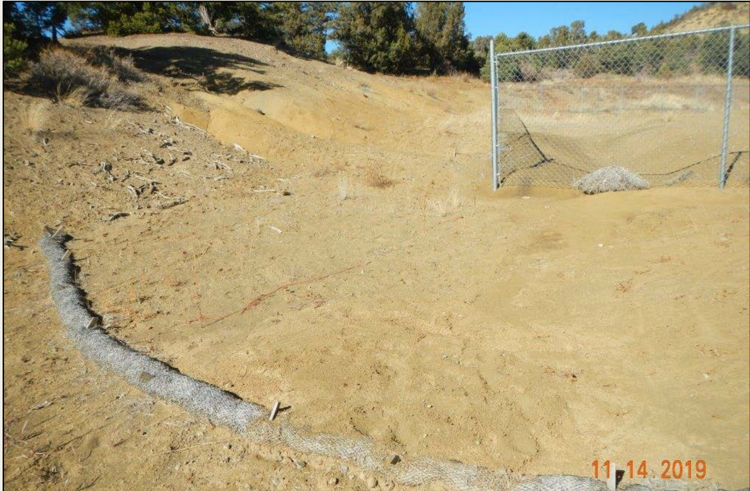
Photo 3. View of area with significant erosion in the southwestern project area. Wattles are full of sediment and are not adequate stormwater controls in this area. Cut slopes are not stabilized and erosional channels are forming on the slopes, and the sediment flows southwest where it discharges from the project area.
