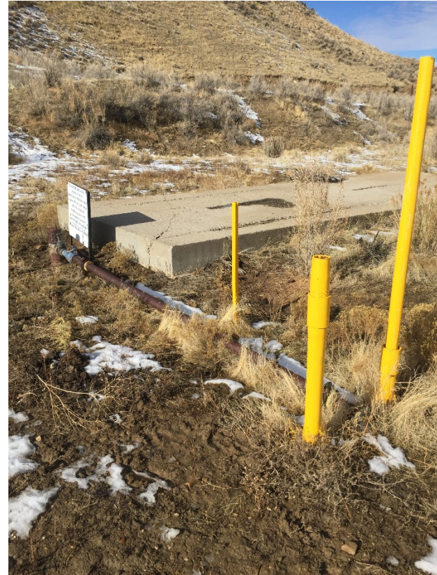
Flowline from wellhead to where it goes underground
