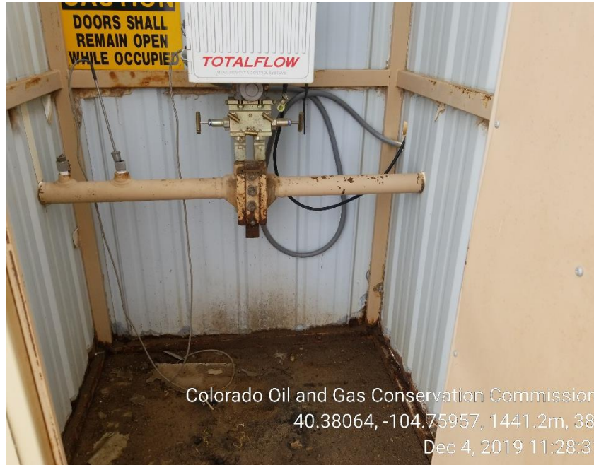
Photo 5: Leak repaired and cleaned up
