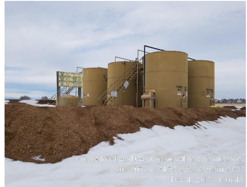
Photo 2: Tank Battery; berm repaired
