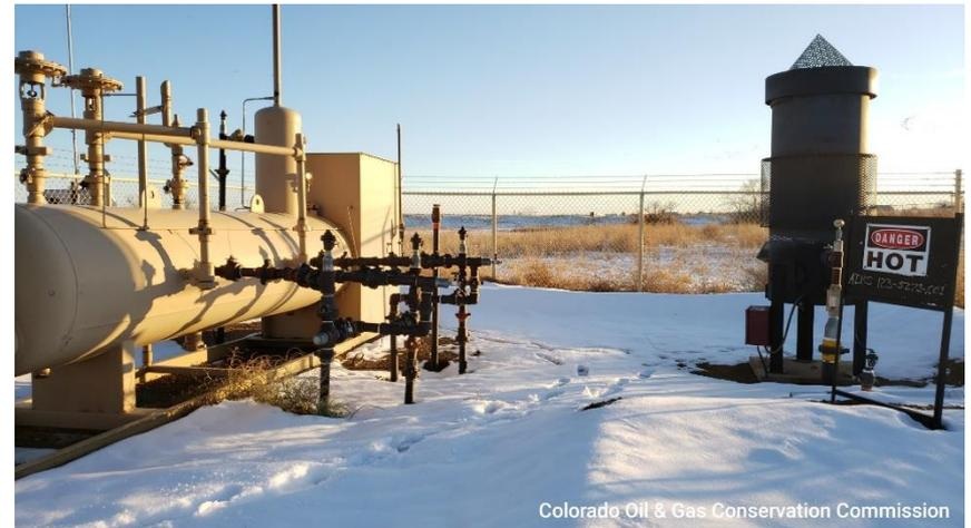
**Photo 3 Gas meter run and pig station**
