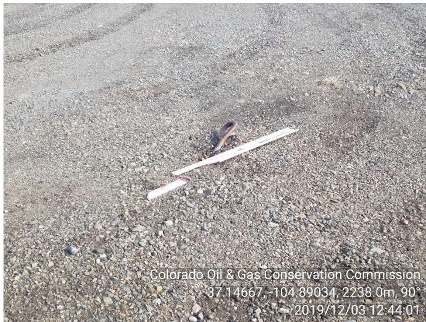
PHOTO 3: GUY LINE ANCHOR MARKER DOWN. INSTALL GUY LINE ANCHOR MARKER IN ACCORDANCE WITH RULE 1003.a. CA DATE 01-3-20.
