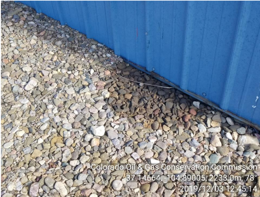
PHOTO 7: OILY IMPACTED SOIL OUTSIDE SOUND WALLS FOR ENGINE SKID FOR X WELL. Remove and dispose impacted material in approved manner, service and maintain equipment and self inspect to prevent recurrence of conditions per 1002.f(2) and 907. CA DATE 01-03-20
