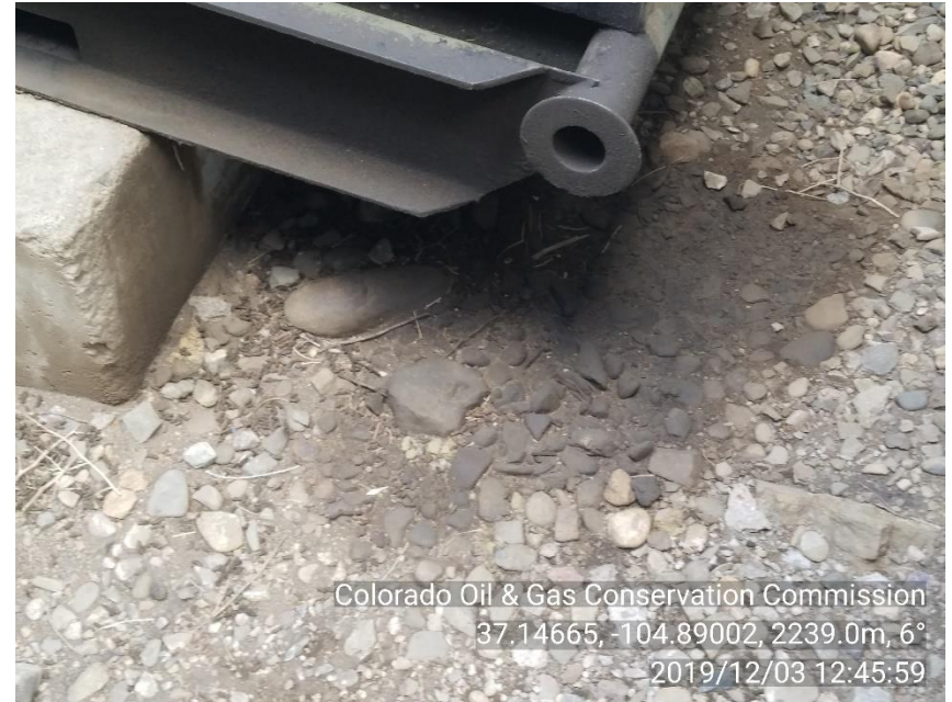
PHOTO 8: OILY IMPACTED SOIL INSIDE SOUND WALLS OF X WELL UNDER ENGINE SKID. Remove and dispose impacted material in approved manner, service and maintain equipment and self inspect to prevent recurrence of conditions per 1002.f(2) and 907. CA DATE 01-03-20
