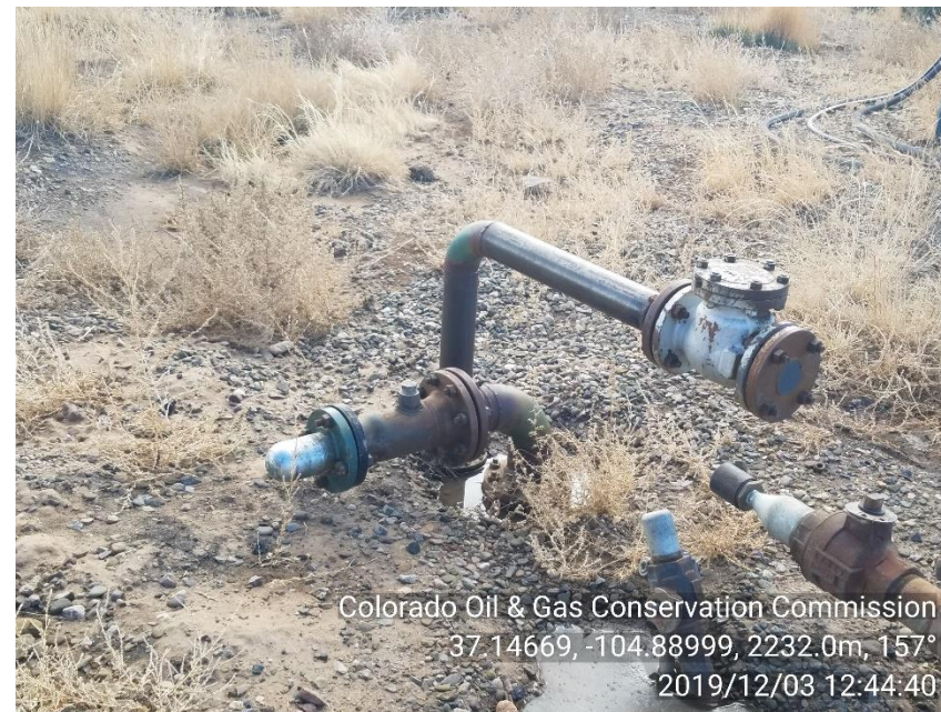
PHOTO 4: TWO UNMARKED UNUSED RISERS NEAR X WELLHEAD. REMOVE UNUSED RISER IN ACCORDANCE WITH NTO AND RULE 603.f. CA DATE 02-3-20.
