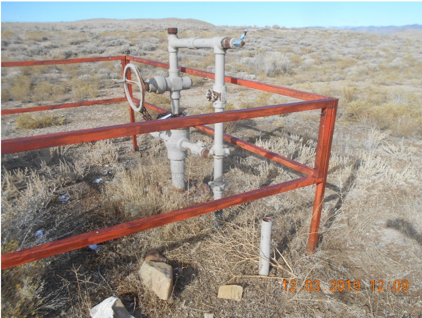
2" flowline riser. Open ended. Not locked out tagged out.
