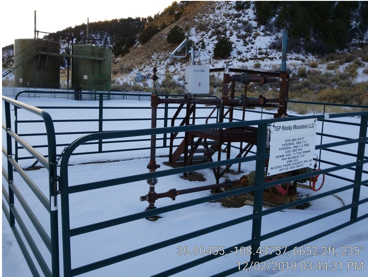
Photo 2. Well head & tank battery.
