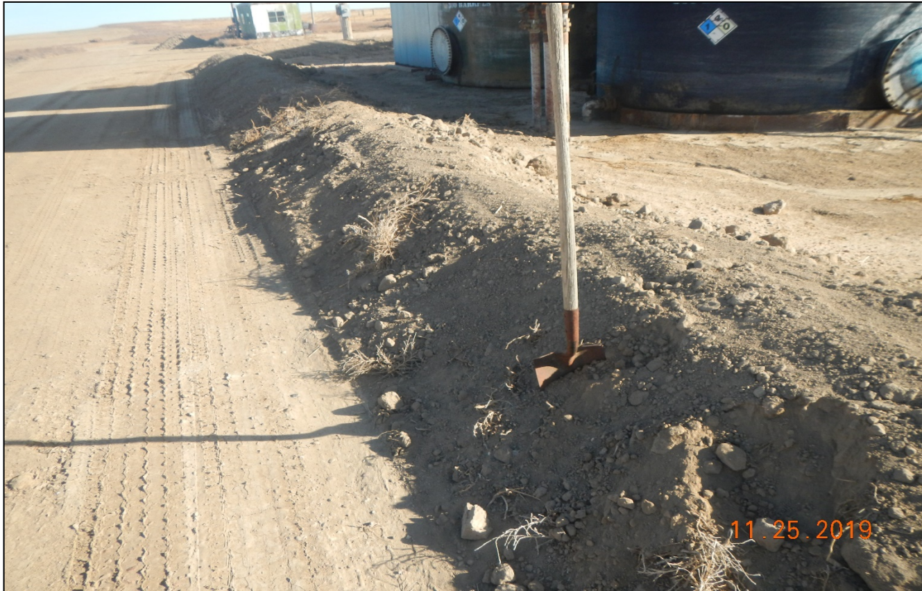
Photo 2. The berm around the tanks have been built up however, soils are loose and not compacted.
