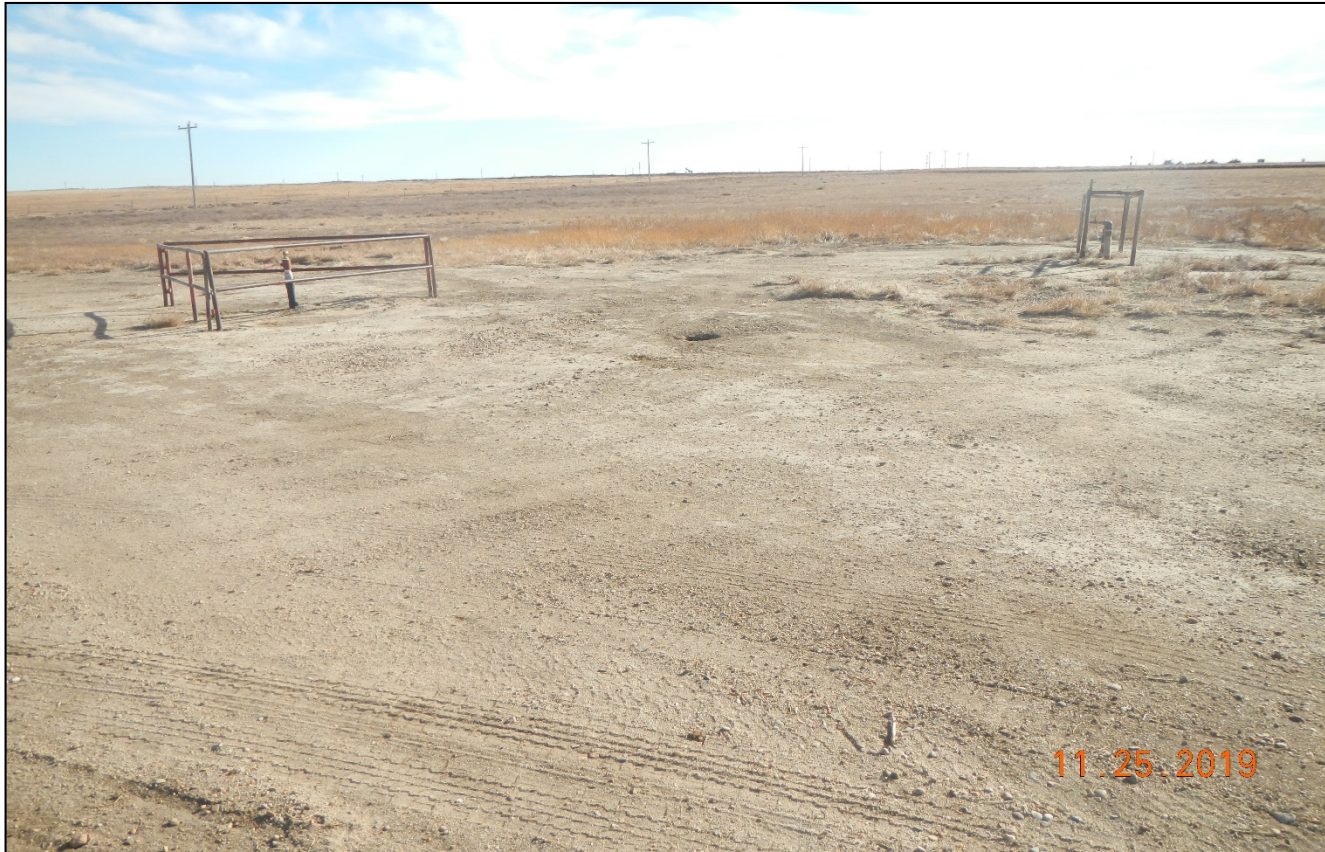
Photo 6. The pipe risers are now protected by a metal fence. The left riser in the photo has LO/TO. The right does not.
