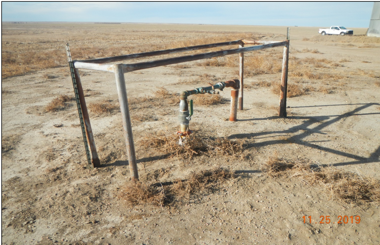
Photo 7. Facing northeast at the south side of the location. This pipe riser has no LO/TO.
