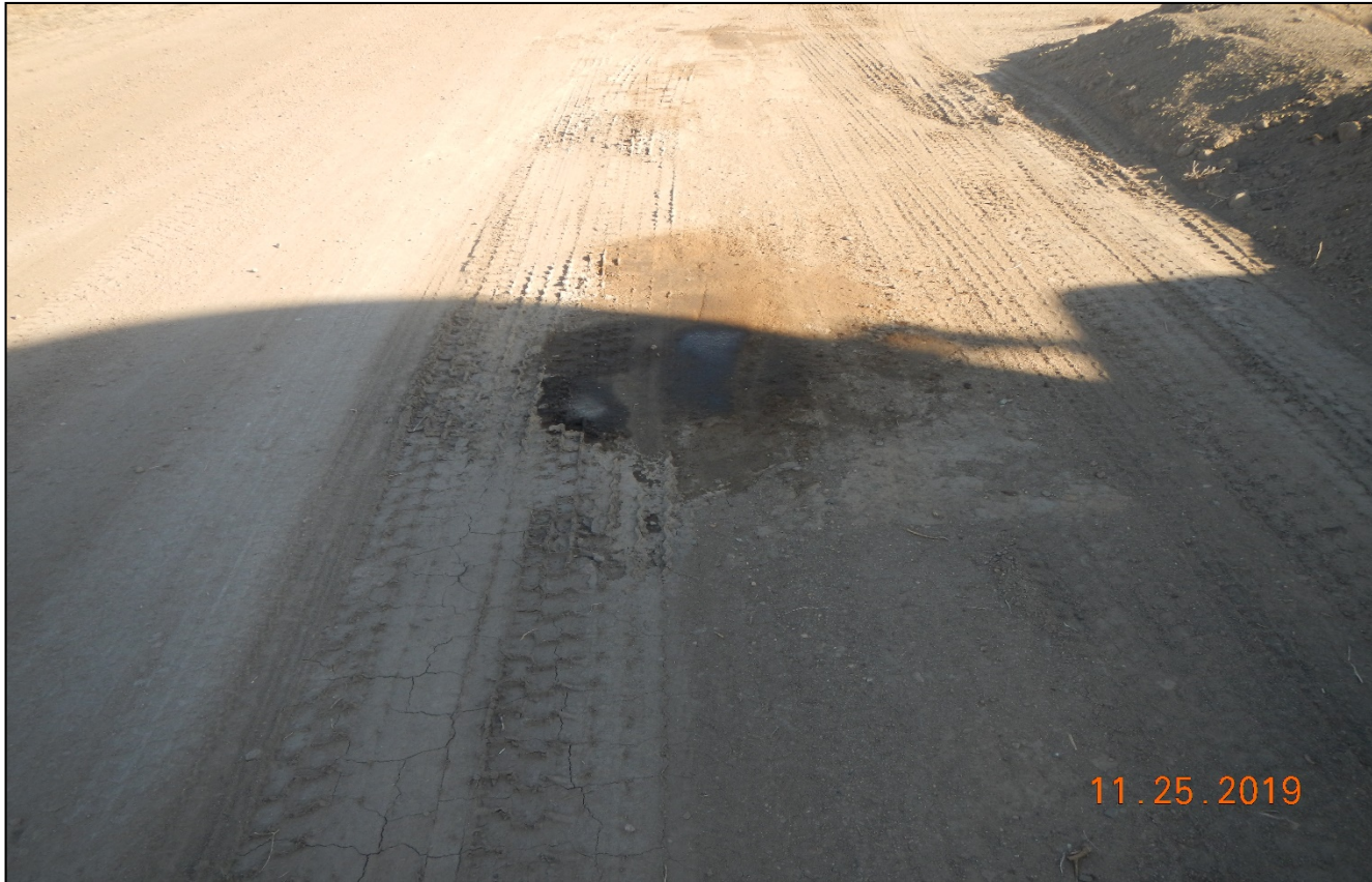
Photo 3. There is oil stained soil on the road surface near the tank battery has not been cleaned up. Approximately 4 ft. x 4 ft. area.
