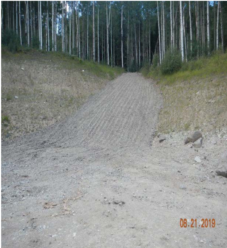
Photo#2: Cuttings were in process of being spread on cut slope .
