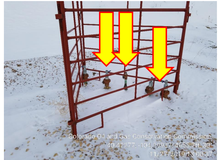
Photo 4 – Unmarked 1" and 2" Risers west of Separators
