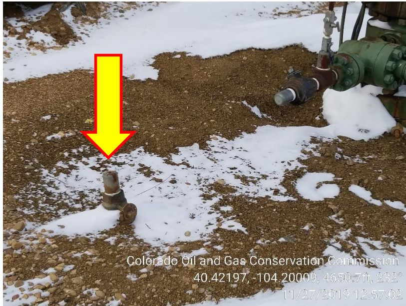
Photo 3 – Unmarked 2" Riser at South Wellhead
