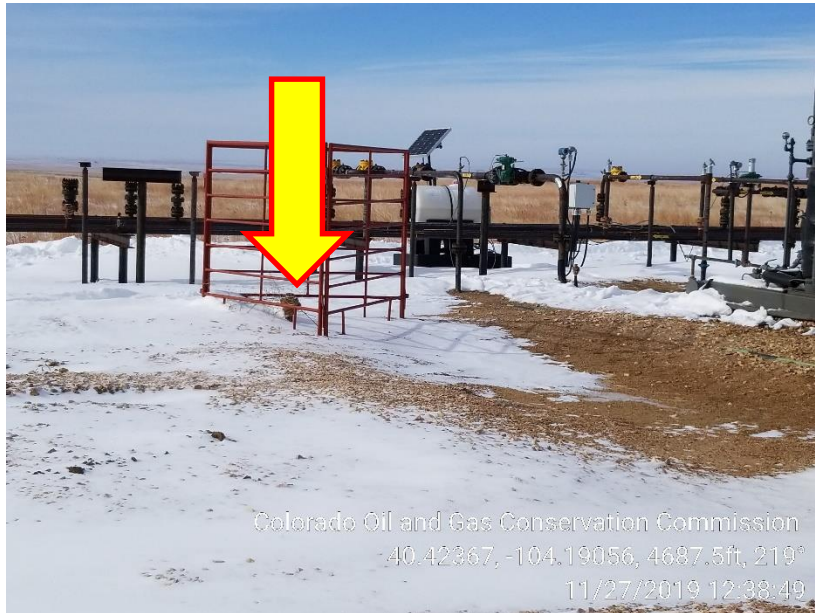
Photo 3 – Unmarked Riser South of Compressor
